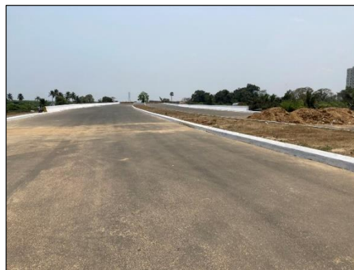
Small-scale infrastructure project under the Program (Construction of a bypass road) (Source: Evaluator)
