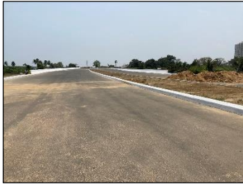
Construction of Bypass Road
