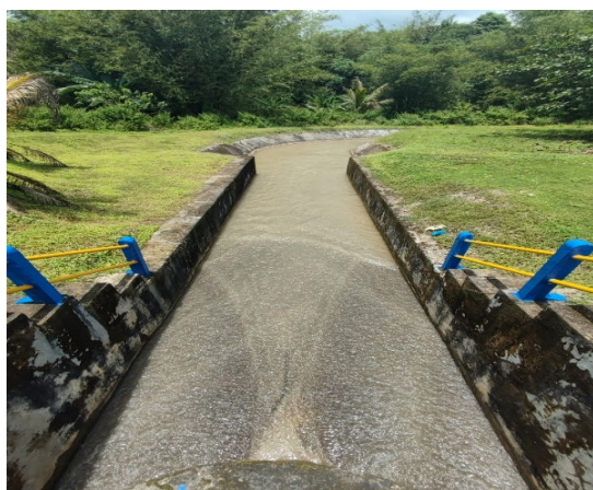
Water Diversion Point from the Intake Weir (Way Apu Subproject)
