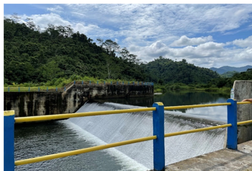
Developed Dam (Tommo Subproject)
