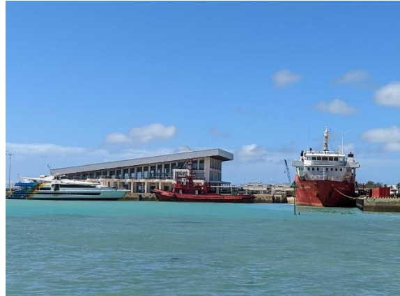
Domestic wharf developed in this project 1 (Source: External Evaluator)
