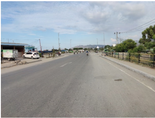
Photo 6: Developed Access Road
