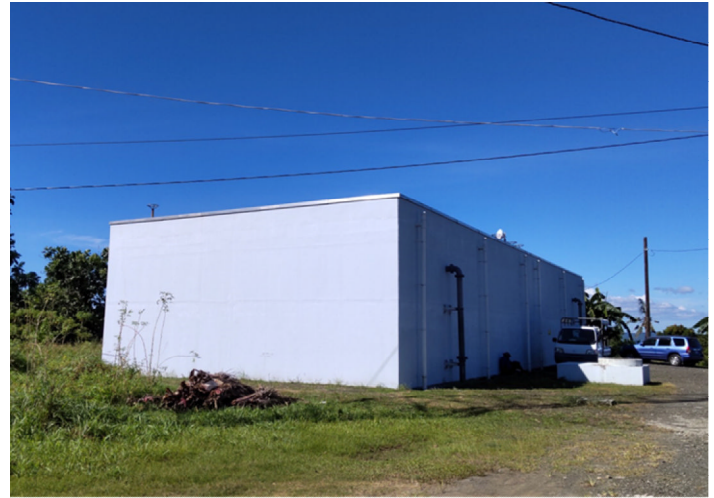
Malakal service tank, newly constructed under this project (source: taken by the evaluator)
