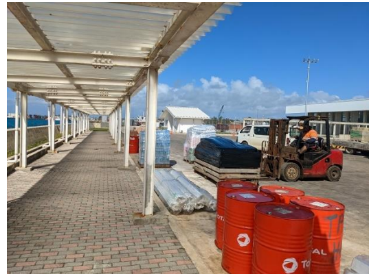
Covered passenger walkway (Photo by External Evaluator)
