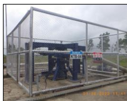
New borehole for demonstration testing (Kedungtuban borehole)
