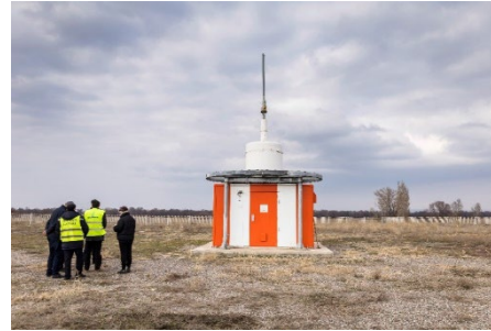
Air Navigation Facilities:, VHF Omni-directional Range (VOR) / Distance Measuring Equipment (DME) (source: JICA)
