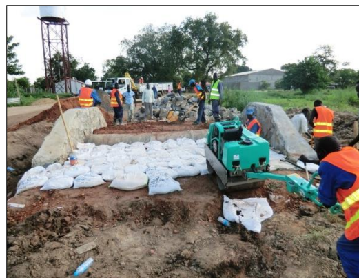
OJT of road repair using sand bags (September 2013) Source: Project Team
