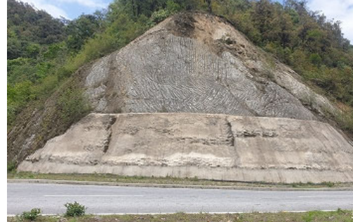
Slope mortar spraying along the access road to Zalamchu Bridge
