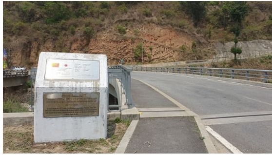
Sidewalk of Chuzomsa Bridge
