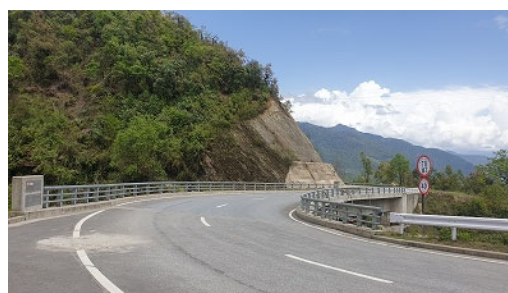
Curving Zalamchu Bridge
