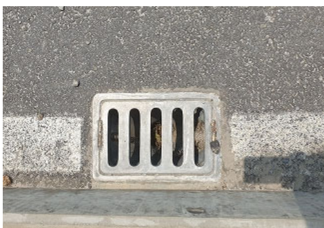
Drainage Outlet of Chuzomsa Bridge
