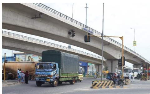
Flyover constructed by the project (photo by the evaluator)
