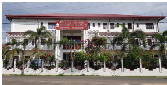
New hospital building at Kaluwanchikuddy BH
