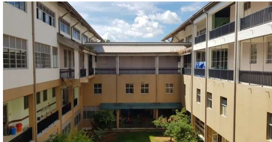
New hospital building at Galgamuwa BH
