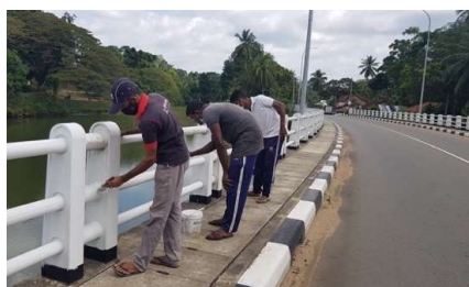
Re-painting of handrails (Denagama bridge)
