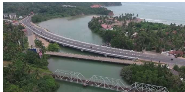
Polwathumodara Bridge, Matara District, Southern Province
