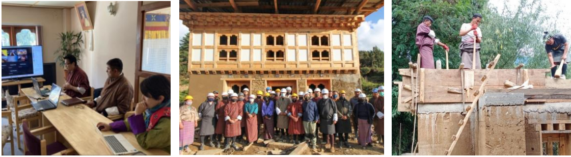
Fig.3-9. Online ToT (left) and Hands-on Training for retrofitting of Dangchu house (middle) and construction of a rammed earth mock wall (right)
