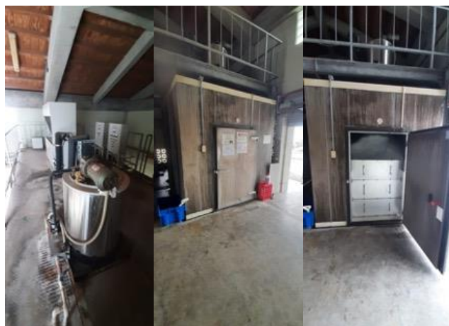
Ice machine, ice storage, and ice inside at Urlings Fisheries Complex
