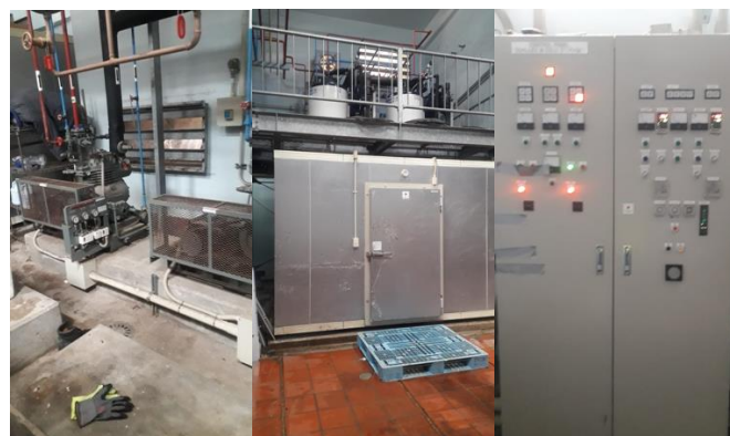
Compressor system, ice maker with drums, and control panels at Grenville Fisheries Complex
