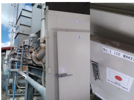
Tower and pump of the evaporative condenser, chill room, and ice maker at Melville Street Fisheries Complex
