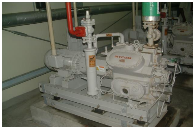
Ice-making machine compressor overhauled in 2016 under this project at Kingstown Fisheries Centre. Photograph taken on August 16, 2021
