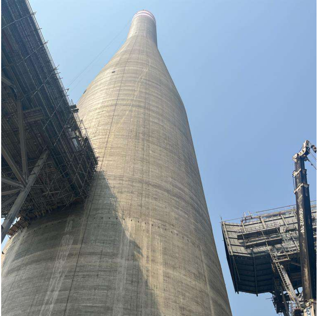
Exhibit 103: MIDI Site Pictures - Chimney (1 of 2)
