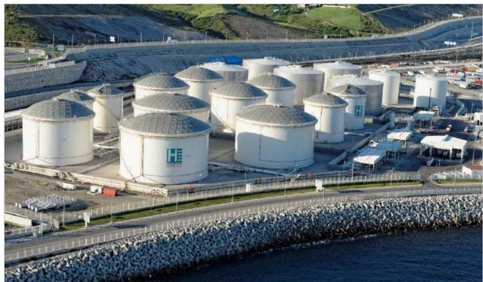
Exhibit 178: Hydrocarbon Terminal at Tanger Med
