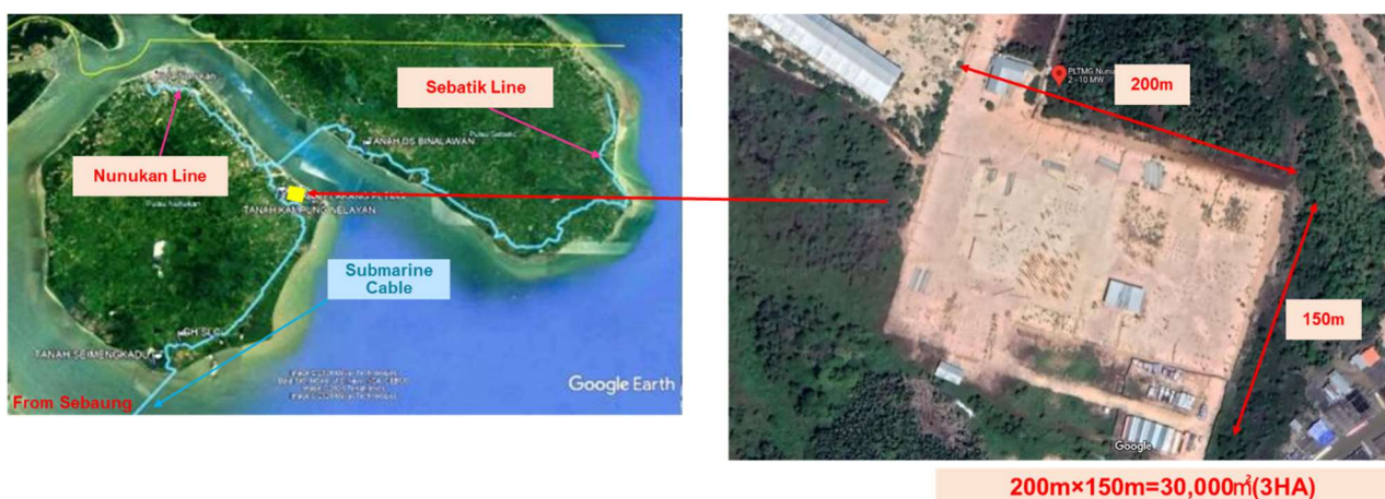
(Source) KYUDENKO Figure 7 Planned site of PLN's gas-engine power plant construction.
