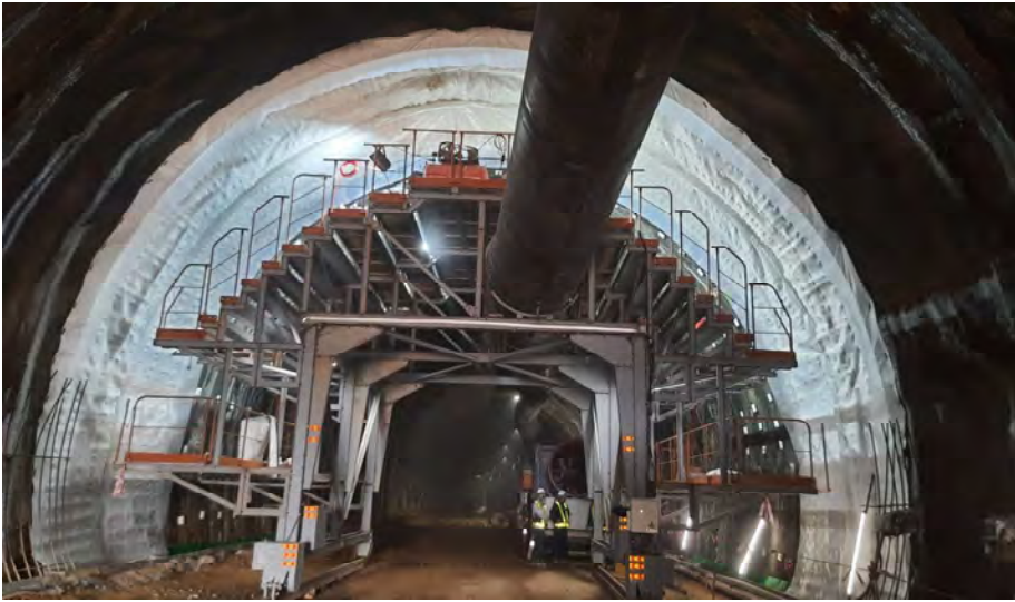
Water Proofing Works at East Main Tunnel
