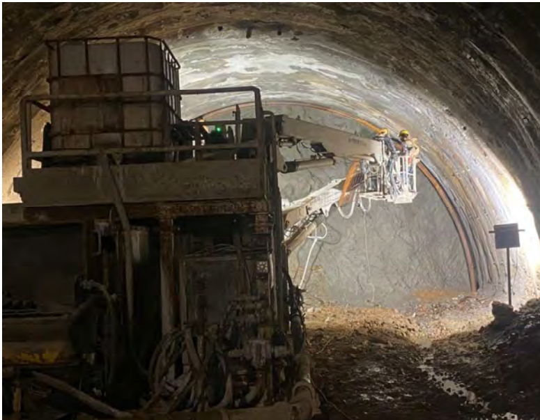
Excavation work completed up to Sta. 2+928.00 in Main Tunnel (East Side)
