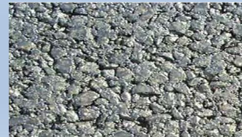
Stone Mastic Asphalt
