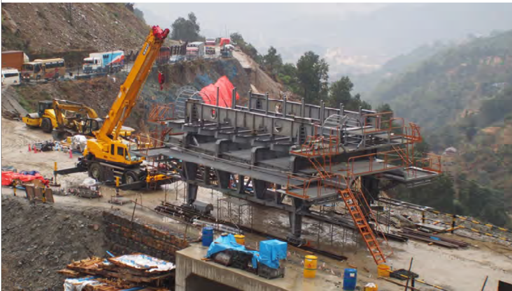
Movable Form Work for Lining
