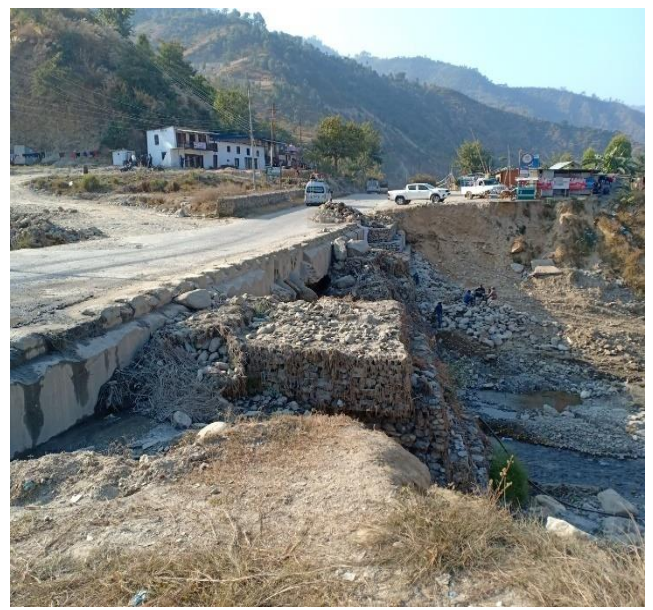
Fig 6: Existing conditions of BP Highway at Bhyakure Khola crossing (Ch. 119+700)
