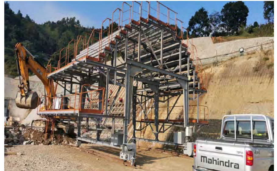
Movable Scaffolding for Water Proofing inside Tunnel Works (East)
