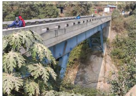
PI Bridge at Narke
