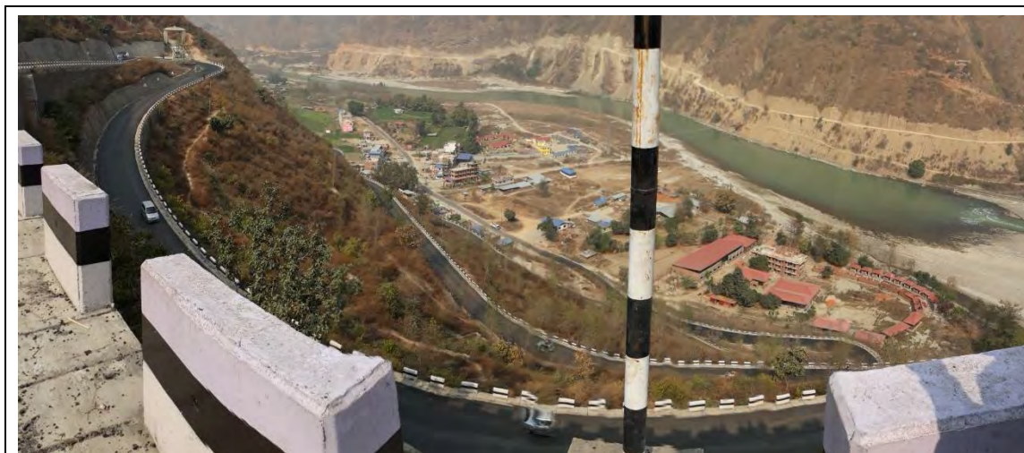
A view of newly constructed pavement at the Mulkot hairpin bend
