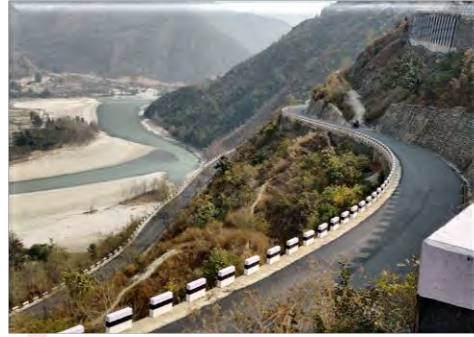
Newly Laid Overlay at ch 94+000
