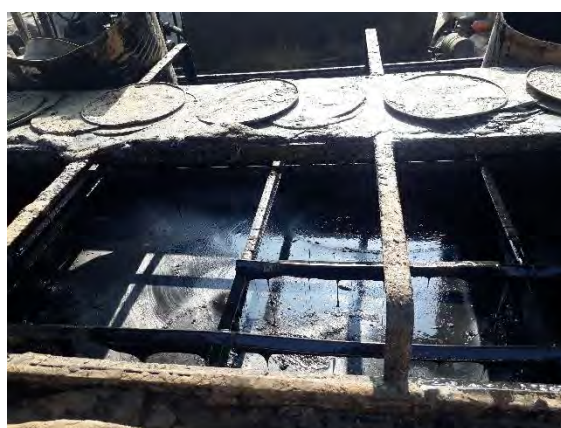
Bitumen stored in the plant
