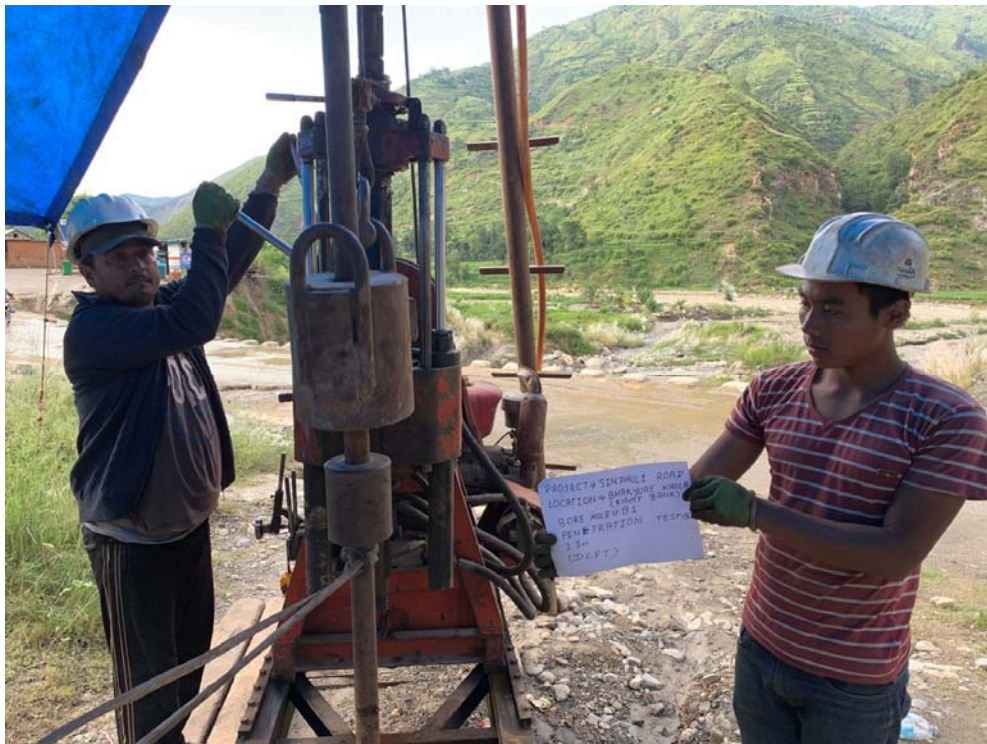
Figure 4: DCPT at borehole B1 (at depth 13 m)
