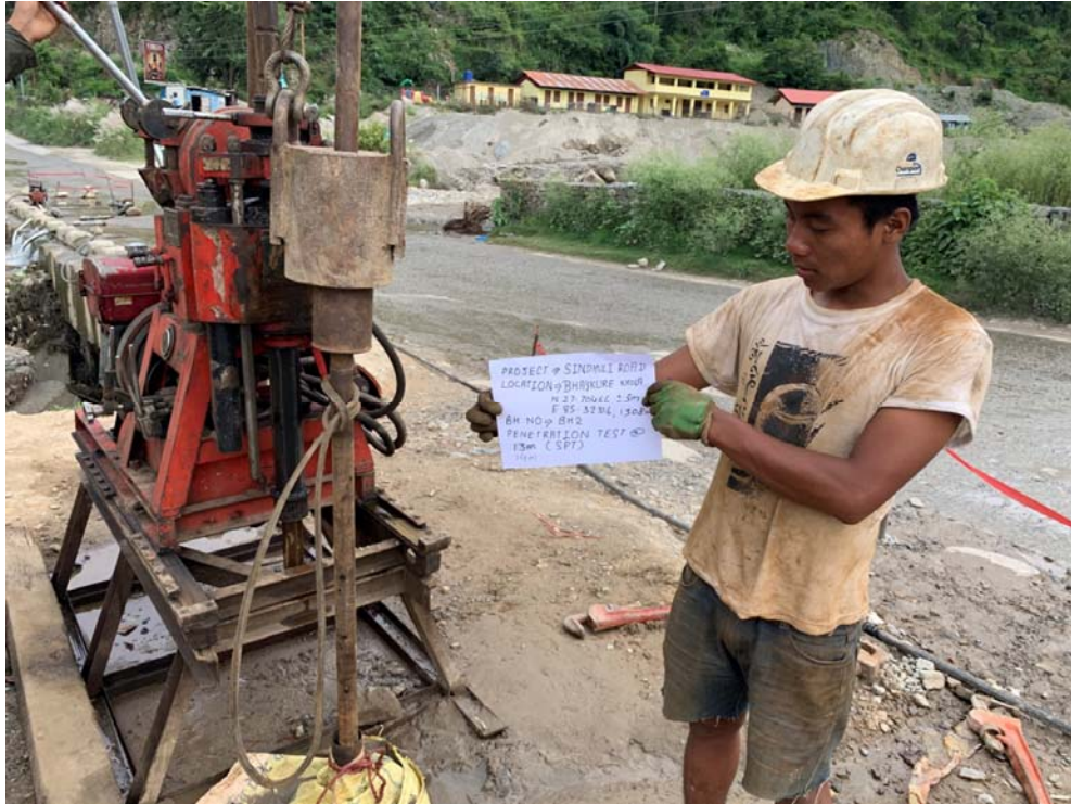
Figure 5: DCPT at borehole B2 (at depth 14 m)
