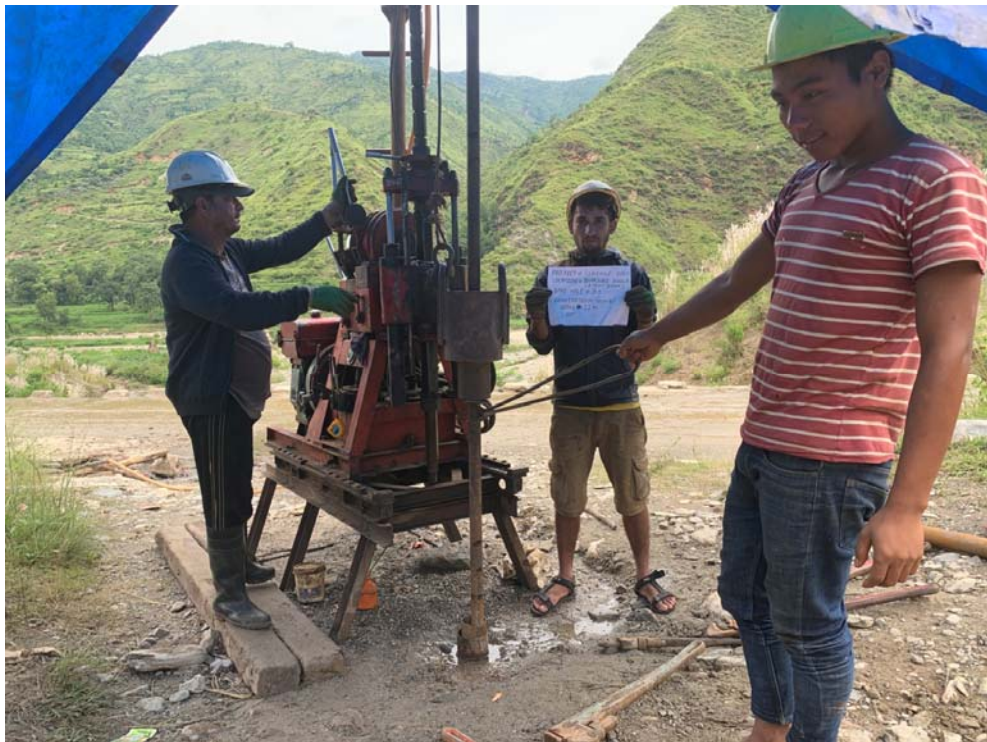
Figure 2: DCPT at borehole B1 (at depth 11 m)
