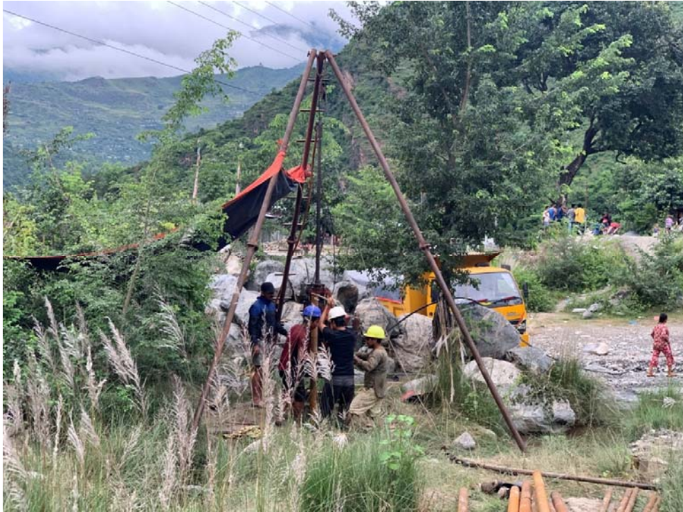
Figure 4: Operating Drill rig at G2
