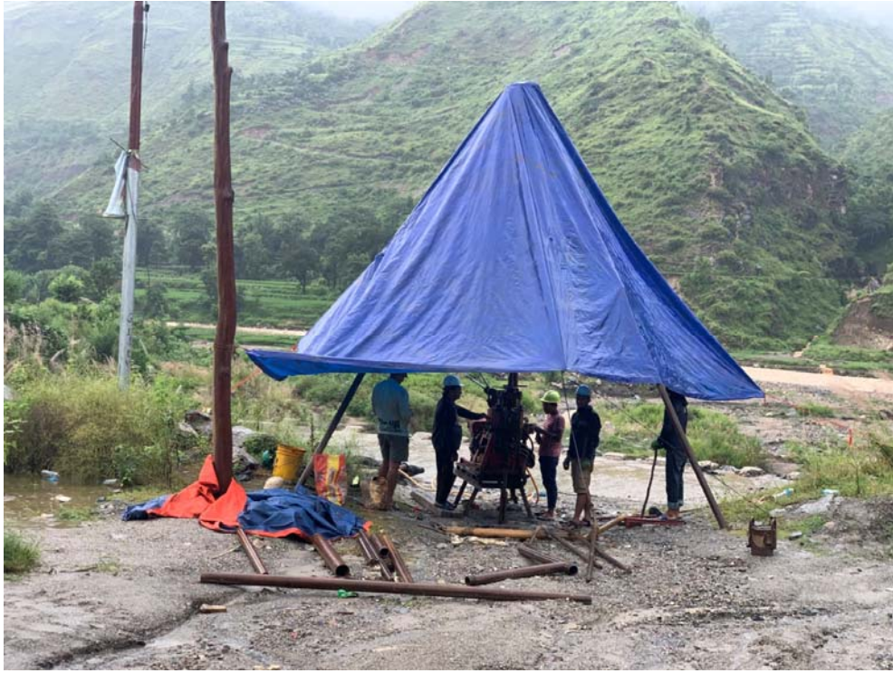
Figure 2: Photo from upstream of Bhyakure Khola at B1
