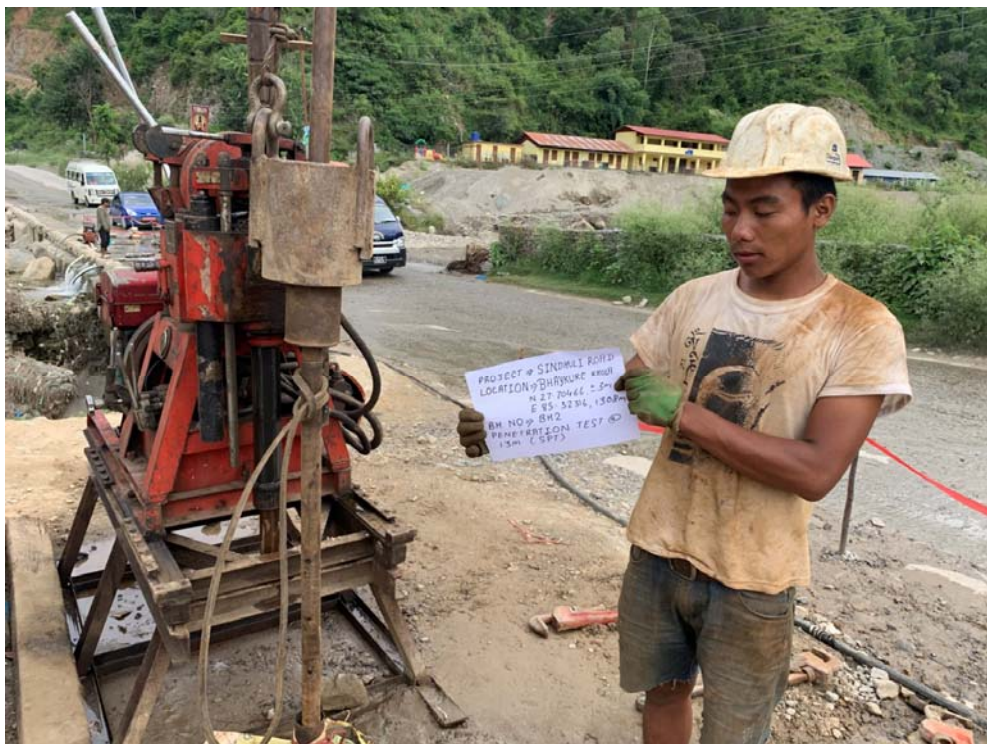
Figure 4: DCPT at borehole B2 (at depth 13 m)
