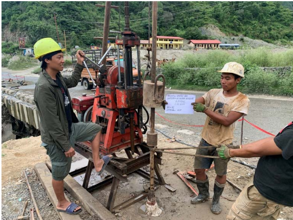
Figure 8: DCPT at borehole B2 (at depth 16 m)
