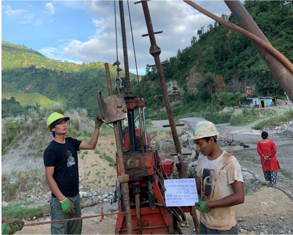
Figure 1: DCPT at borehole B2 (at depth 10 m)
