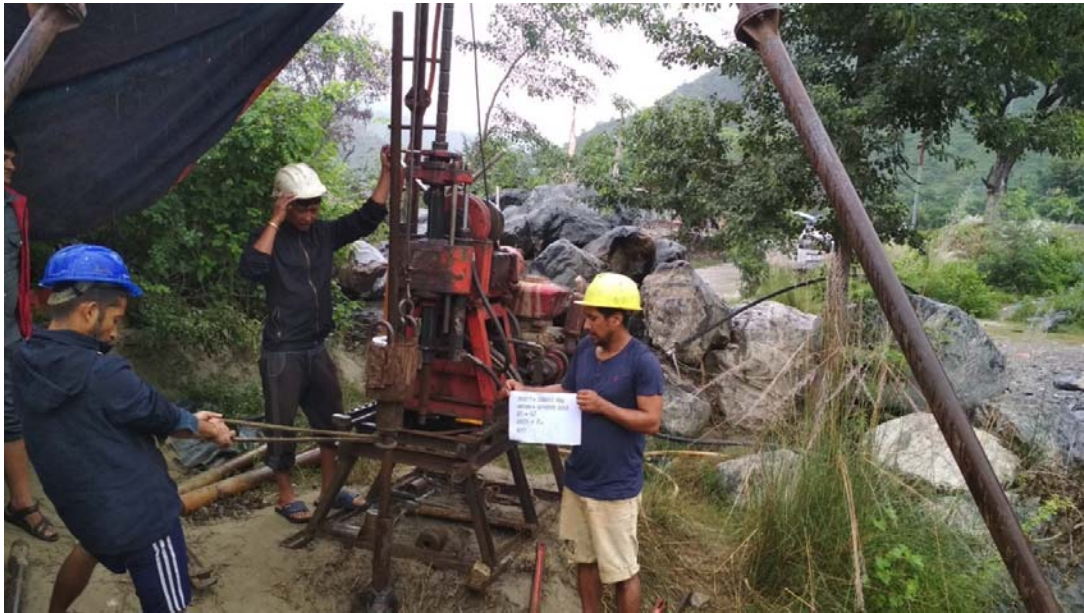
Figure 5: DCPT at borehole G2 (at depth 15 m)
