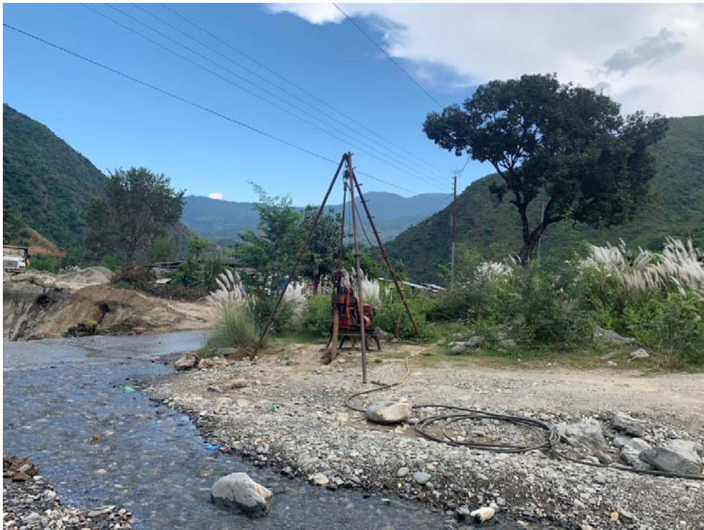
Figure 5: Drill rig before operation at G1
