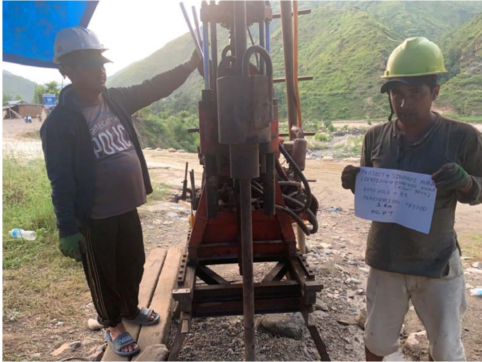
Figure 7: DCPT at borehole B1 (at depth 16 m)
