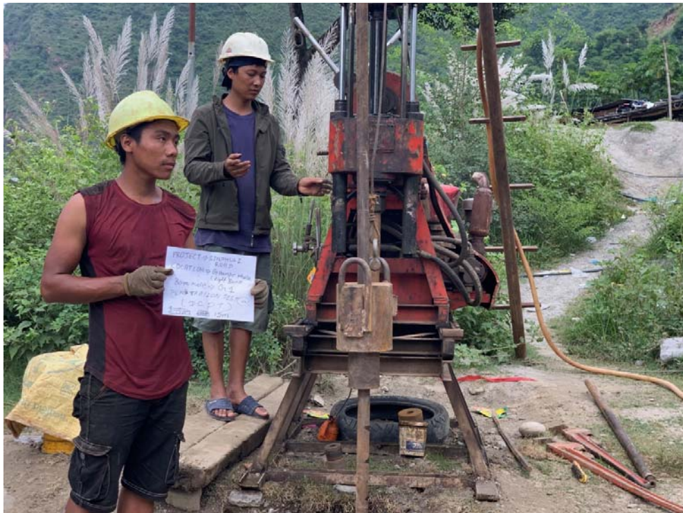
Figure 6: DCPT at borehole G1 (at depth 15 m)
