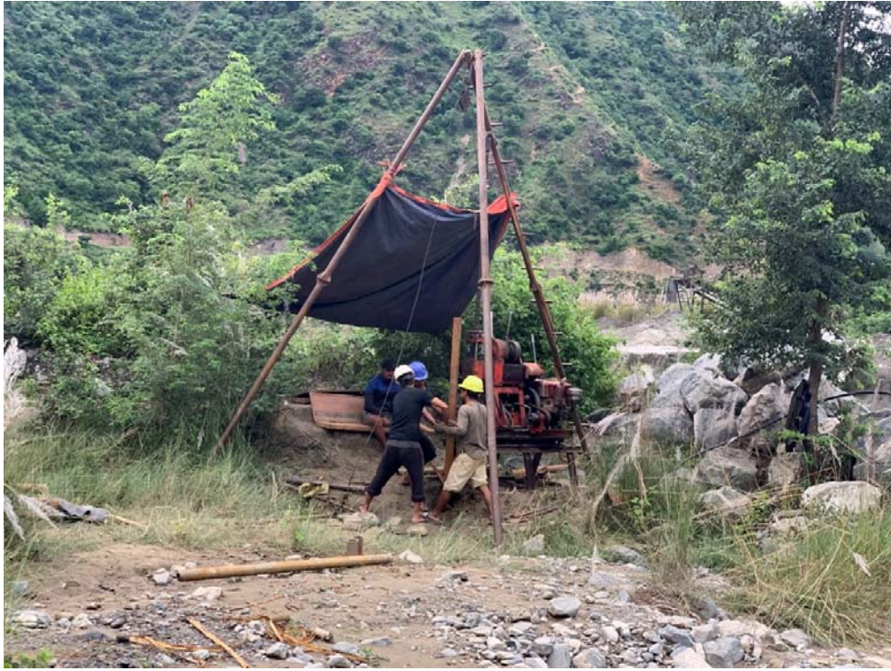
Figure 2: Photo from upstream of Ghyampe Khola at G2
