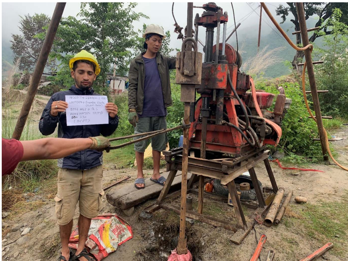
Figure 3.1 Field photograph of DCPT test
