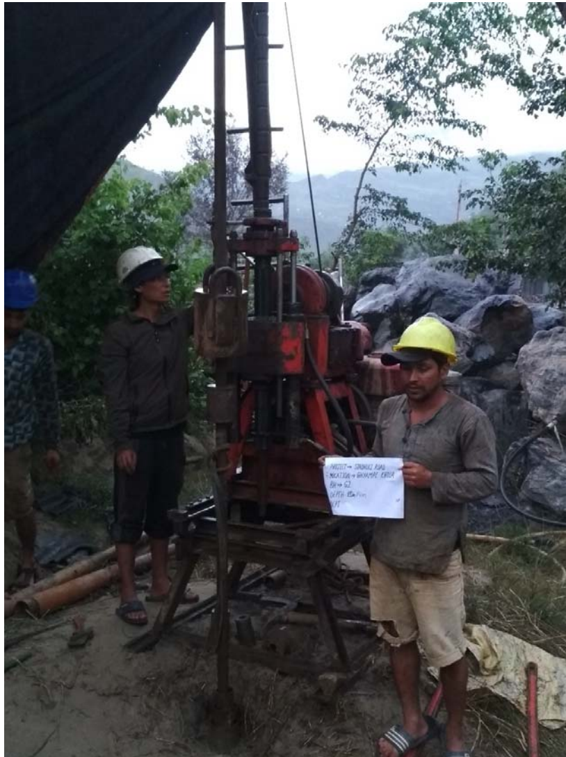
Figure 4: DCPT at borehole G2 (at depth 14 m)
