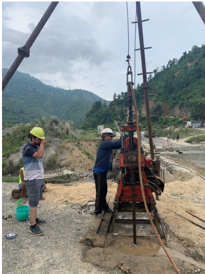
Figure 5: Operating Drill rig at B2
