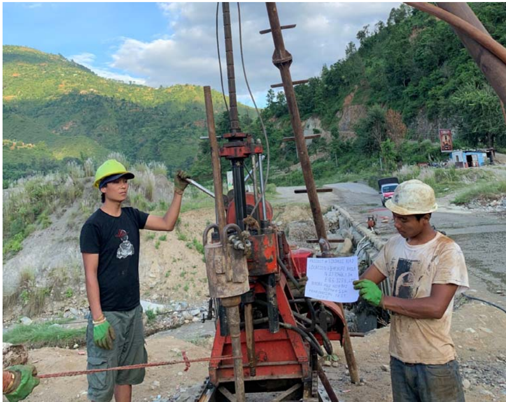
Figure 2: DCPT at borehole B2 (at depth 11 m)
