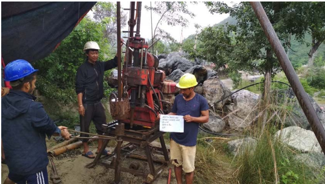
Figure 6: DCPT at borehole G2 (at depth 16 m)
