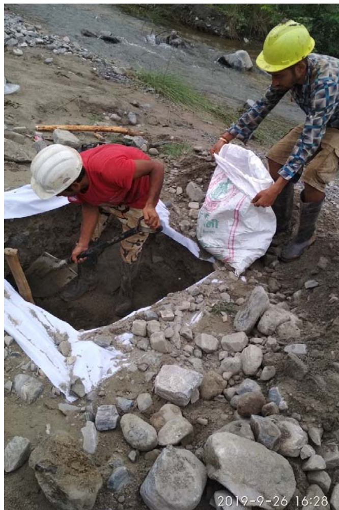
Figure 6: Digging of Test Pit at Ghyampe Khola
