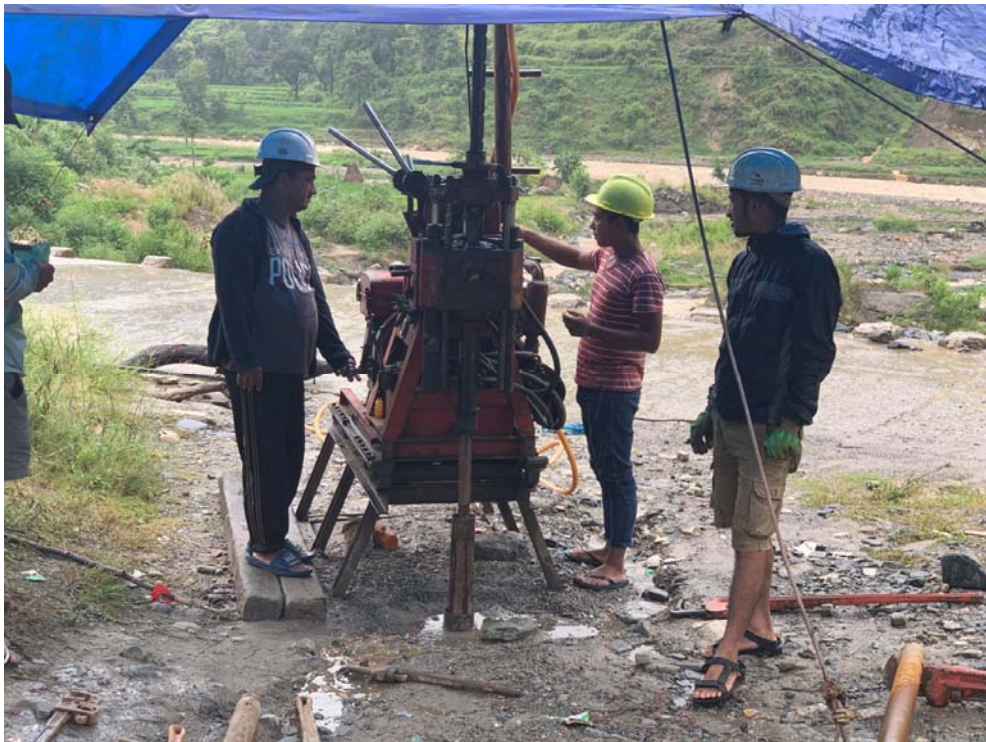
Figure 5: Operating Drill rig at B1
