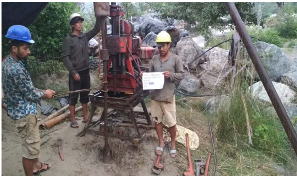
Figure 2: DCPT at borehole G2 (at depth 12 m)
