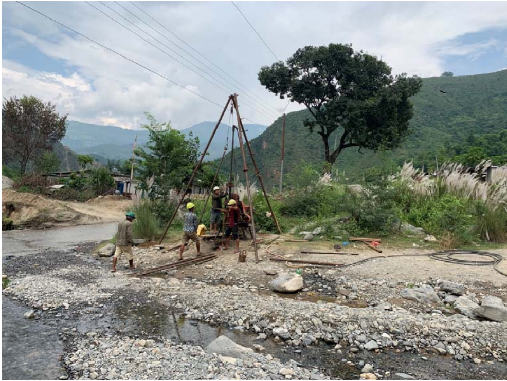
Figure 6: Operating Drill rig at G1
