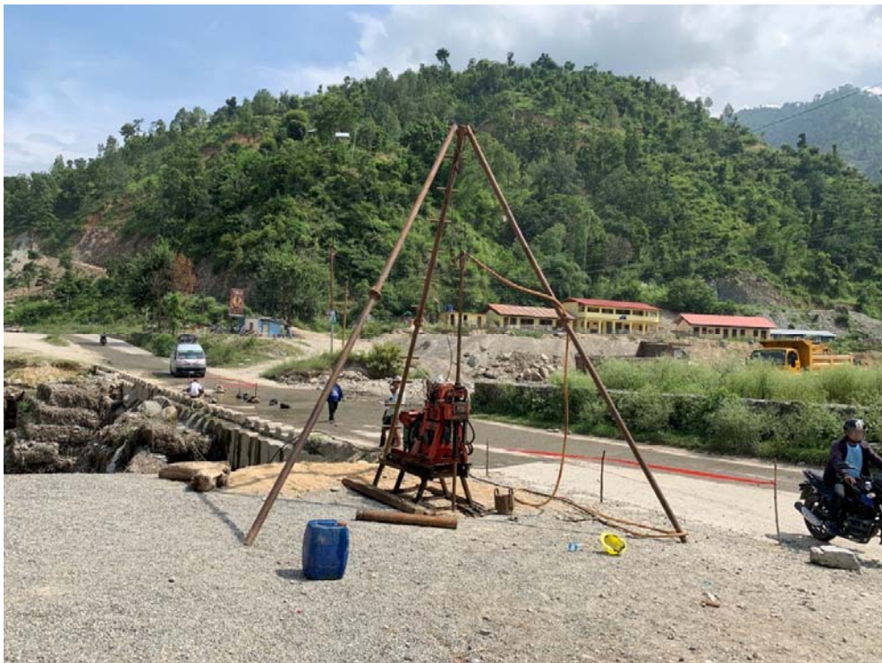
Figure 4: Drill rig before operation at B2
