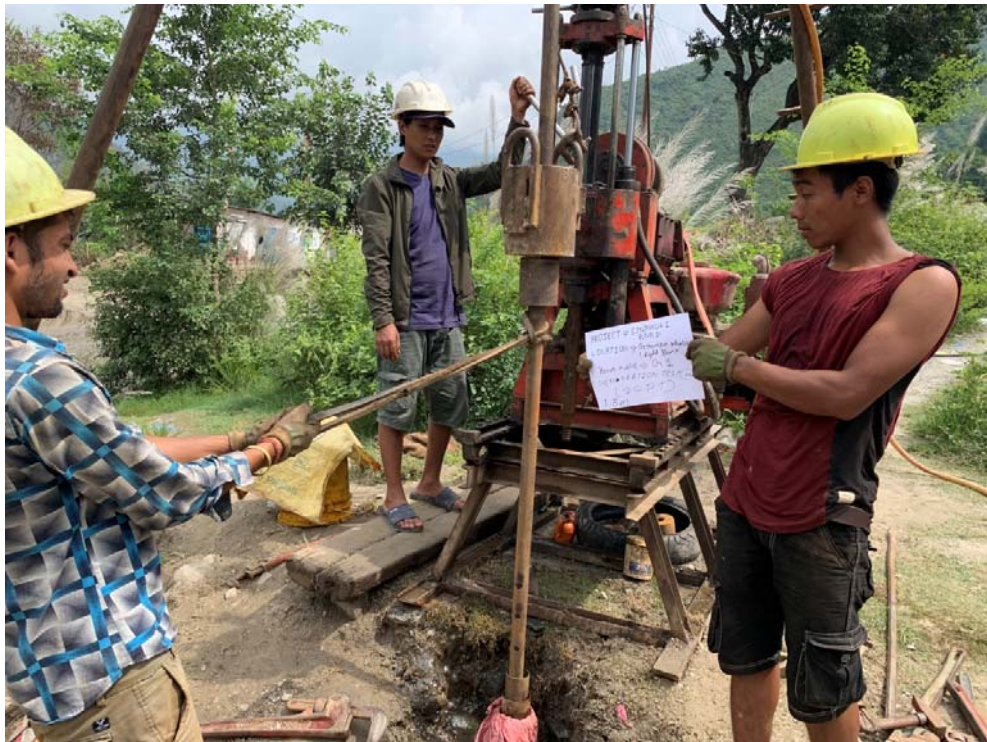
Figure 4: DCPT at borehole G1 (at depth 13 m)
