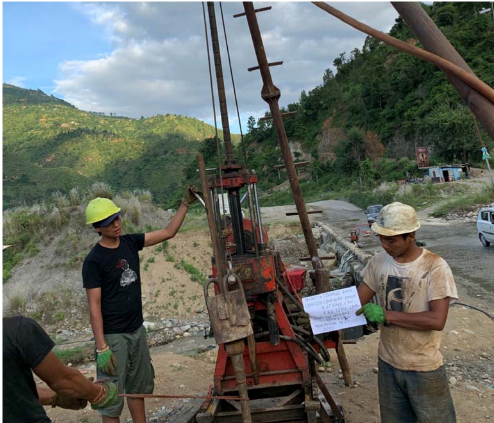
Figure 3: DCPT at borehole B2 (at depth 12 m)
