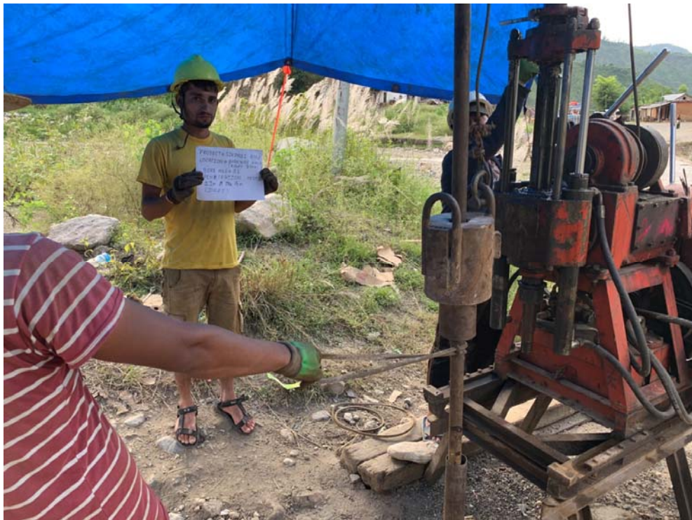
Figure 6: DCPT at borehole B1 (at depth 15 m)
