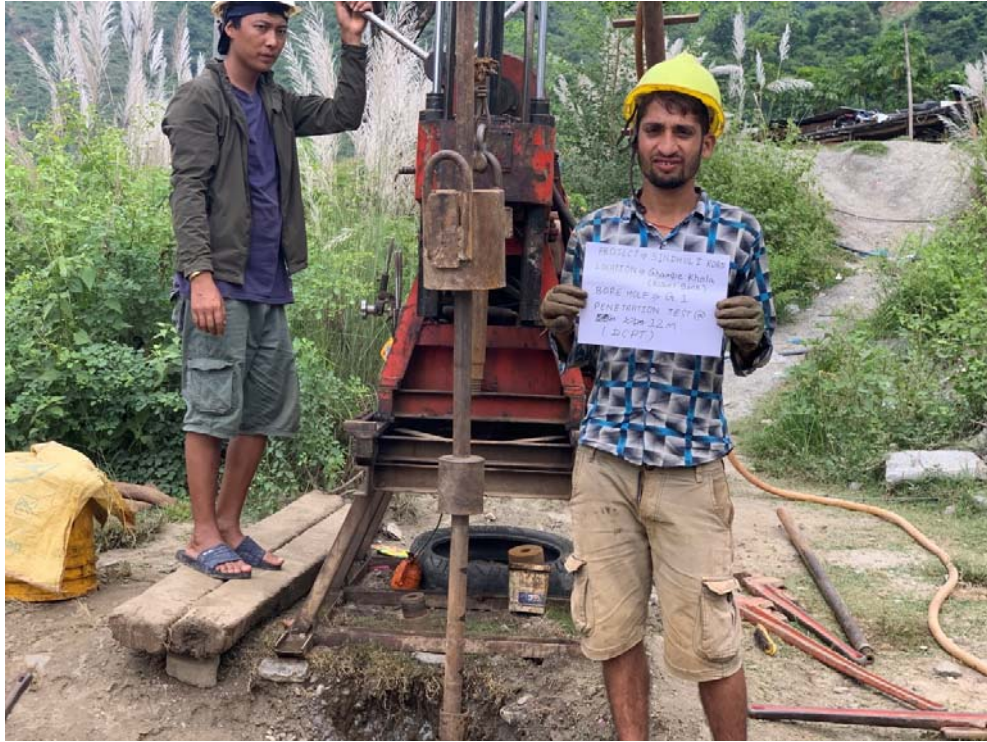
Figure 3: DCPT at borehole G1 (at depth 12 m)
