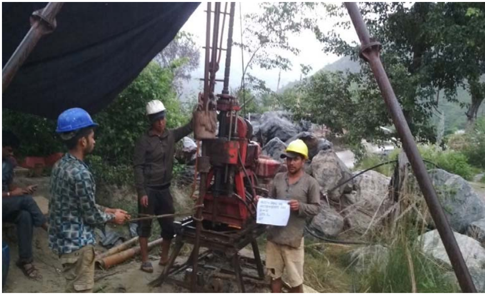
Figure 3: DCPT at borehole G2 (at depth 13 m)
