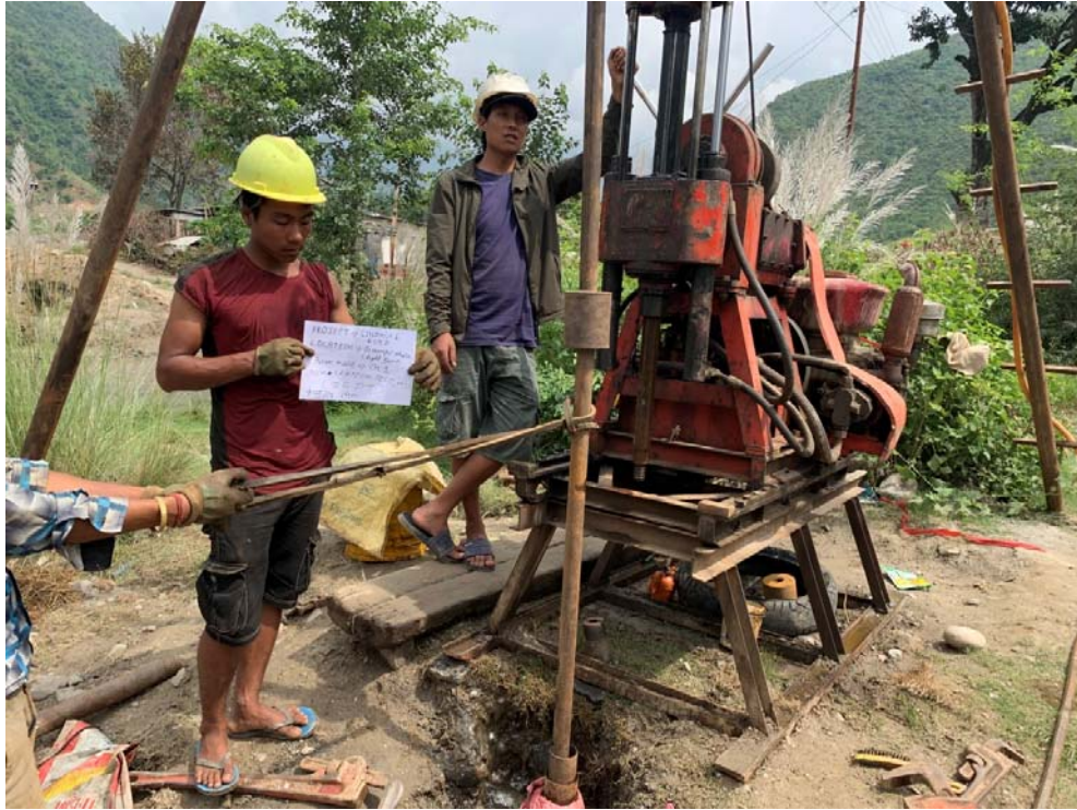
Figure 5: DCPT at borehole G1 (at depth 14 m)
