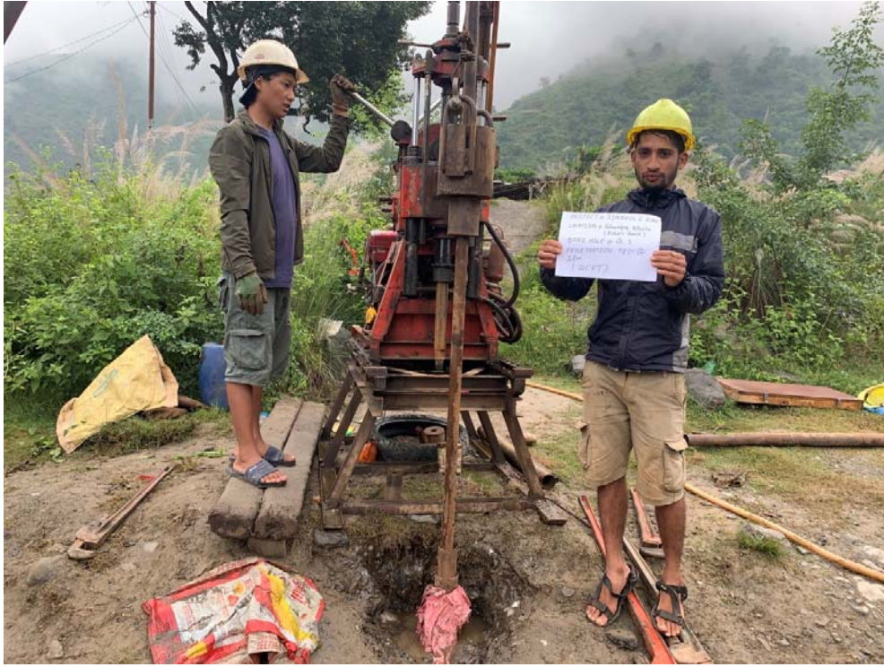
Figure 1: DCPT at borehole G1 (at depth 10 m)
