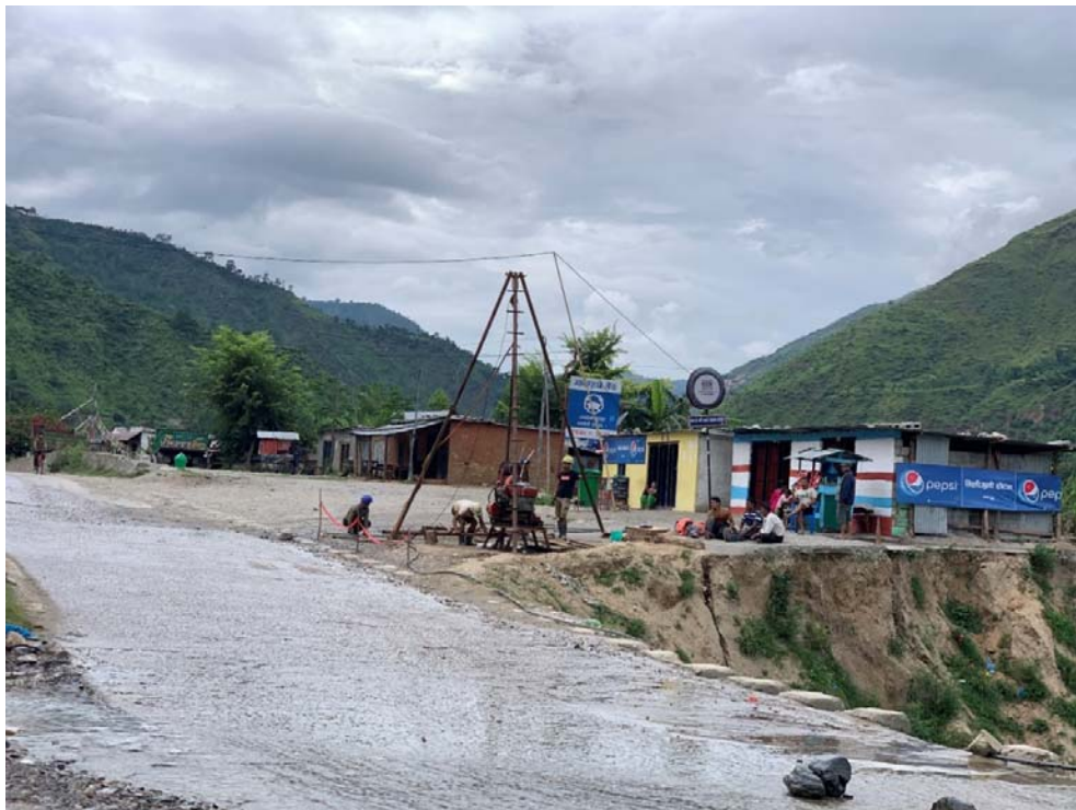
Figure 6: Operating Drill rig at B2
