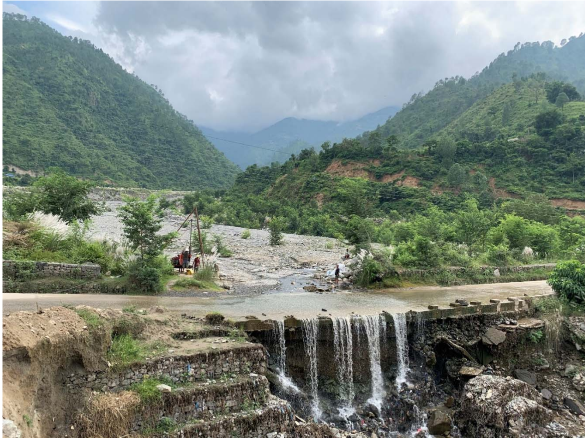
Figure 4.2 Site photograph at Ghyampe khola.
