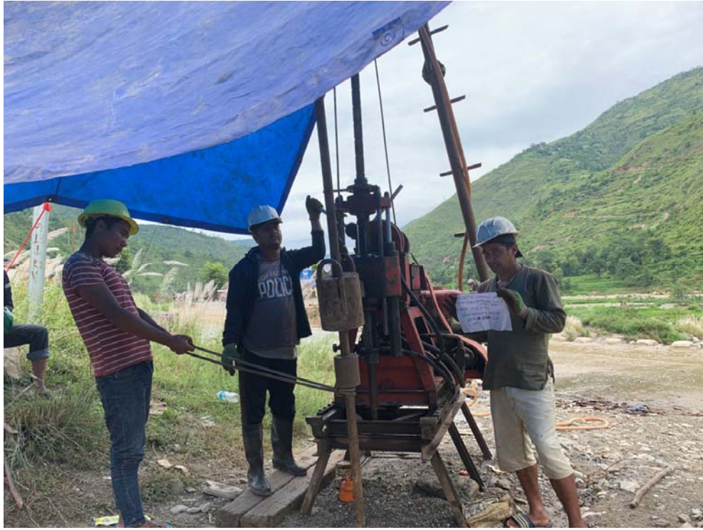
Figure 3: DCPT at borehole B1 (at depth 12 m)
