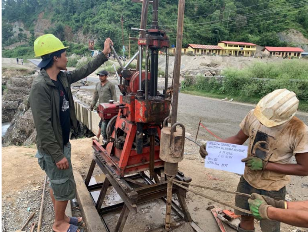
Figure 7: DCPT at borehole B2 (at depth 15 m)
