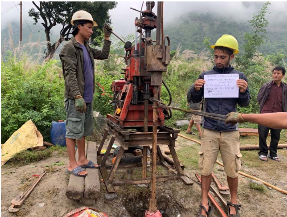
Figure 2: DCPT at borehole G1 (at depth 11 m)
