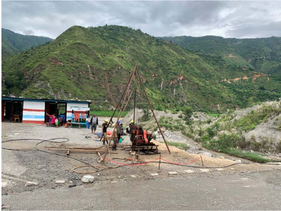
Figure 1: Photo from upstream of Bhyakure Khola at B2
