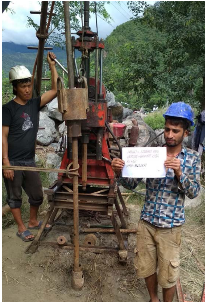
Figure 1: DCPT at borehole G2 (at depth 11 m)
