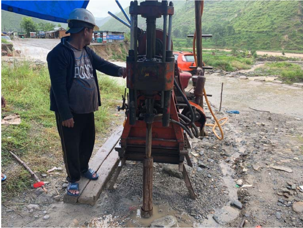
Figure 4: Operating Drill rig at B1
