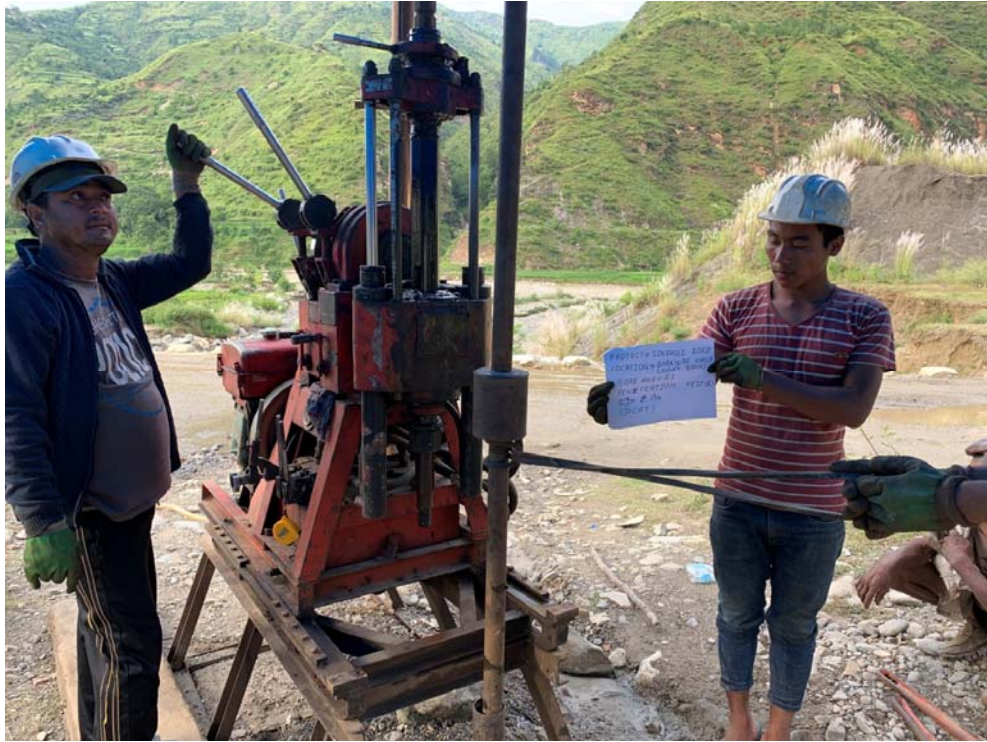
Figure 5: DCPT at borehole B1 (at depth 14 m)
