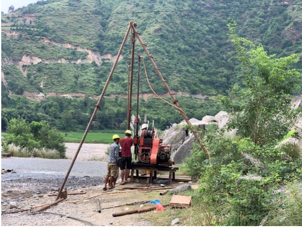
Figure 2: Photo from upstream of Ghyampe Khola at G1
