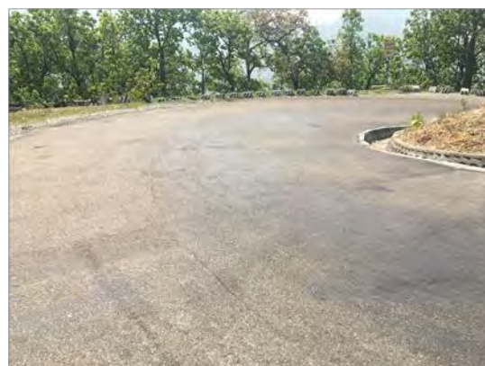
Asphalt Concrete Pavement
