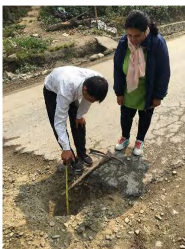
Visual site inspection at Sec. IV of Sindhuli Road
