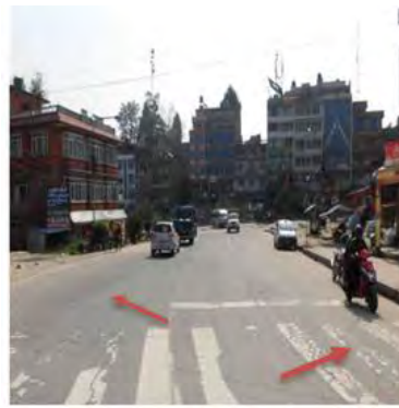
Alligator Crack Near Dhulikhel
