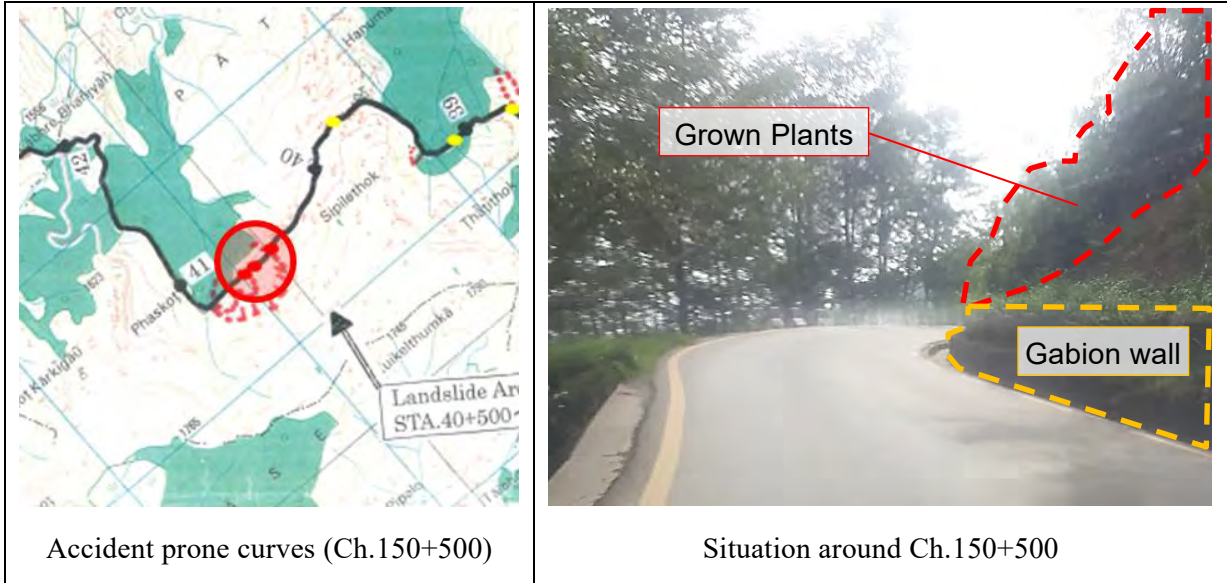
Figure 4-35 Example of Recommended Site for Removal of Plants 1
