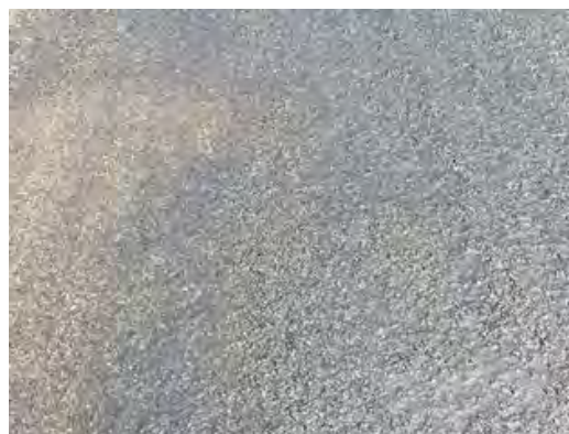
After Applying Slurry Seal
