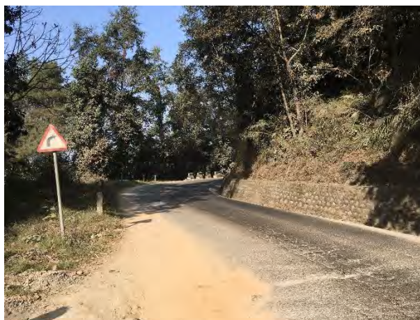
Figure 4-29 Typical Situation of the section from Ch.152+000 to Ch.158+400
