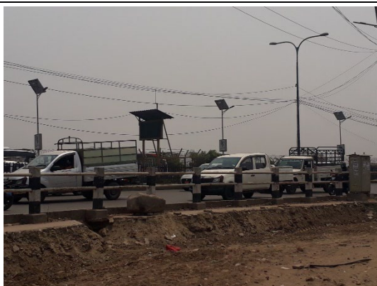
Road widening work and a view of RIB at Koteshwor
