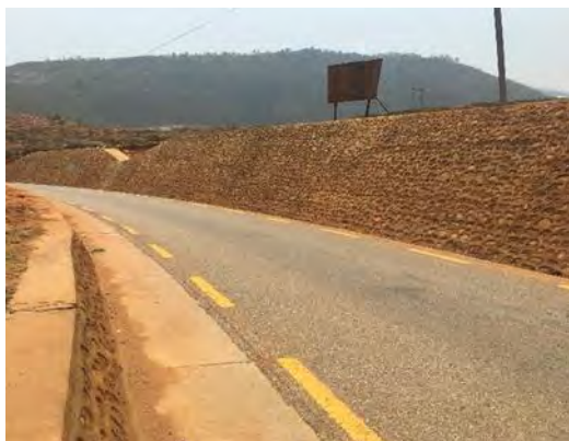
Good condition of DBST
