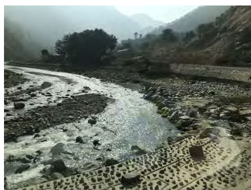
Figure 4-28 Example of Well-Constructed Revetment
