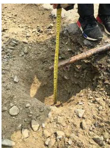
Pavement thickness and subgrade condition
