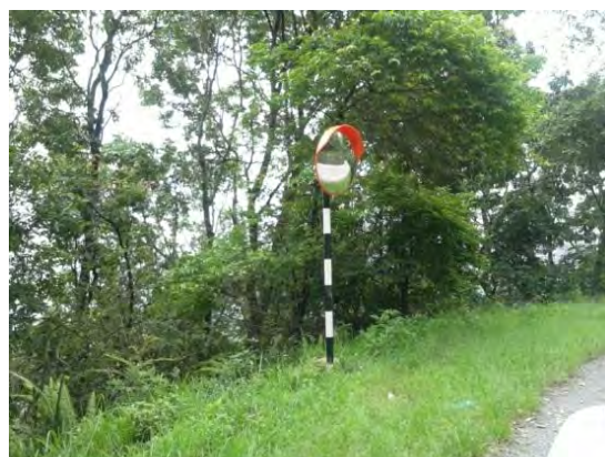
Curve mirror installation on sharp bend
