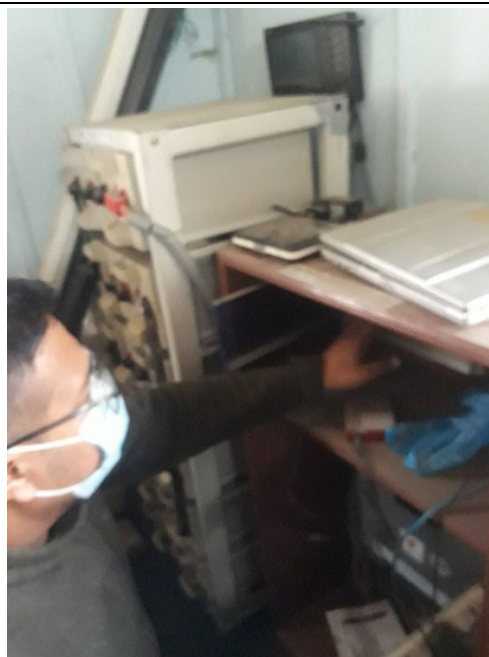
Checking the equipments at the rainfall station
