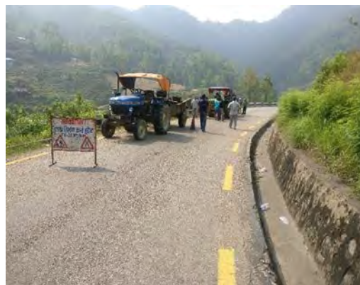
Patching work done on DBST
