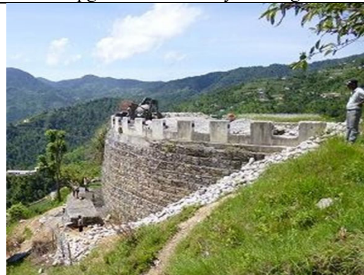
Strengthening Gabion Wall
