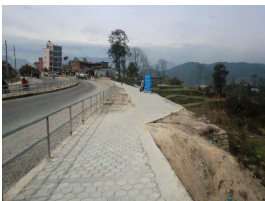
Construction of footpath at high traffic section
