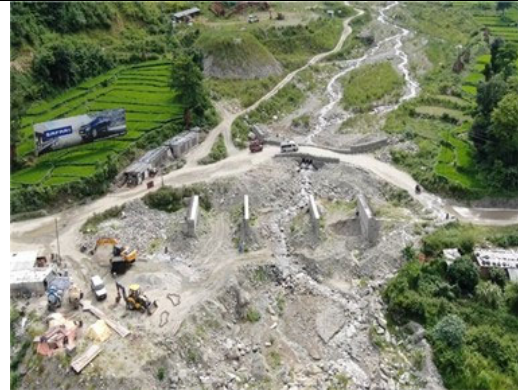
Upgrade of causeway to bridge
