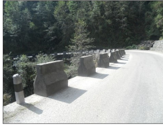
Provision of concrete block
