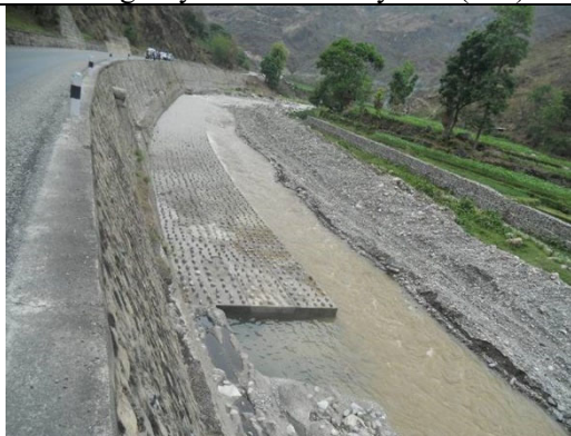
Retaining Wall Foot Protection
