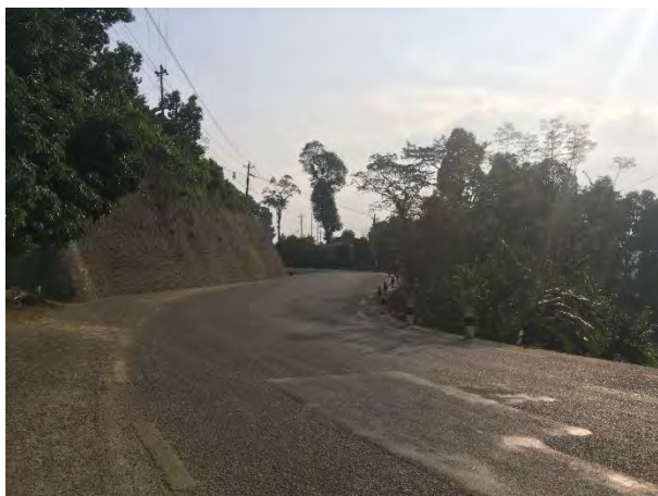
Figure 2-25 Both Side Structure Part in Sindhuli Bazar Area
