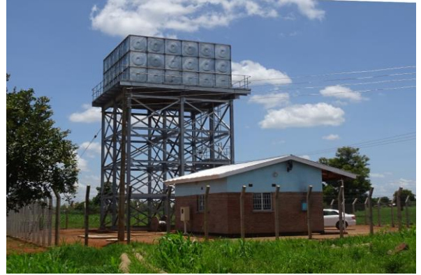
Water tank at Santhe market centre in Kasungu constructed by the project
