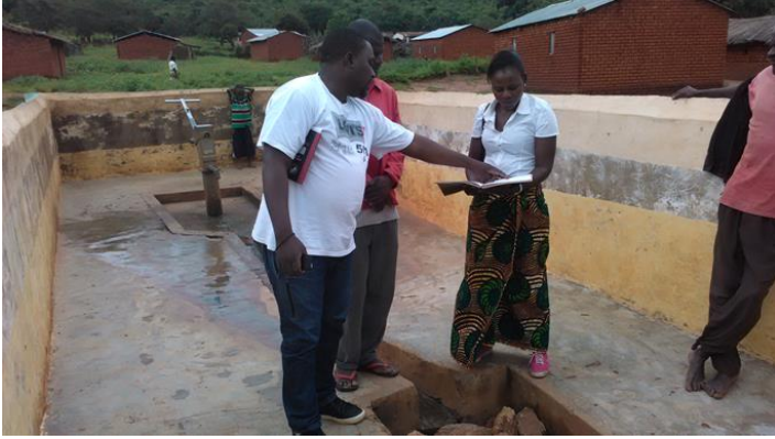
Molosiyo No. 2 Water Point in Mchinji, one of the boreholes constructed by the project. WPC has benefitted from the O&M training during the project.
