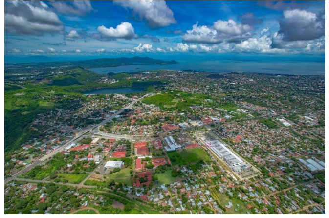
South-North view of the overpass "Las Piedrecitas"
