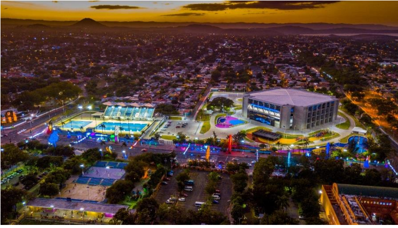
Alexis Arguello Sports Center and the Michelle Richardson Swimming Pool Complex constructed by the Urban Park Development Project
