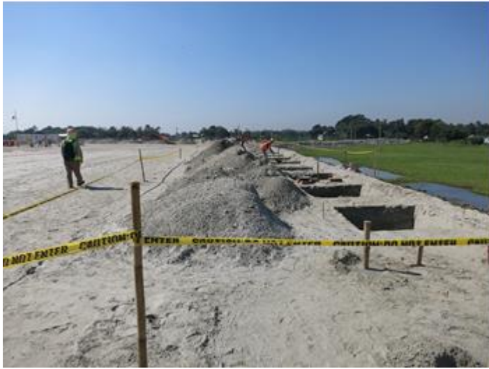
Construction site in the Bangladesh Special EZ
