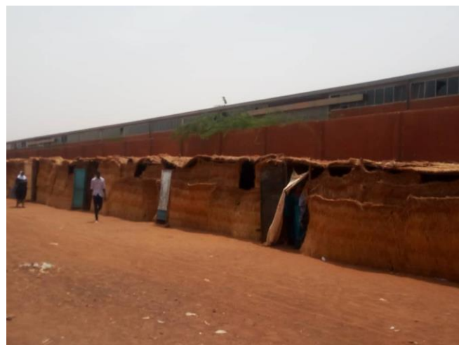
"15 Thatched Classrooms" constructed by CGDES in Pays Bas 1 & 2 Primary Schools
