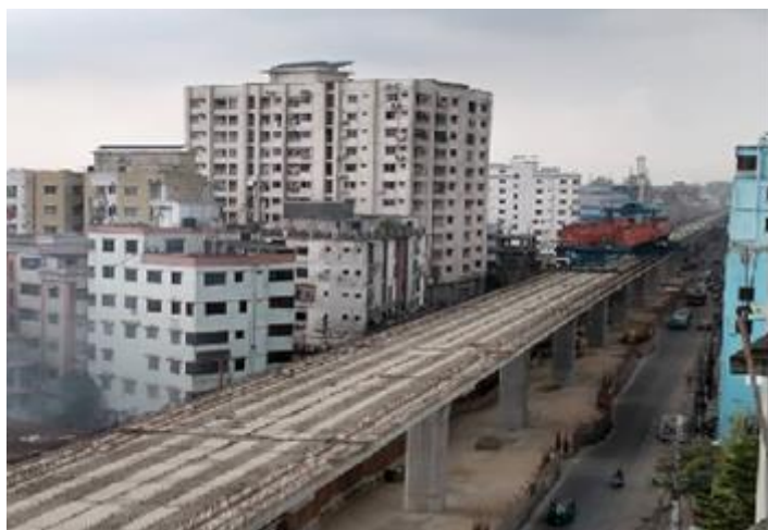
MRT Line 6 construction of elevated section near Kazipara Mirpur
