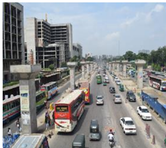
BRT Line 3 construction of piers near Shahjalal International Airport
