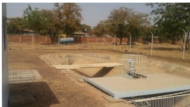
The pilot high-speed algal channel wastewater treatment plant in the campus of Kamboinsé, 2iE
