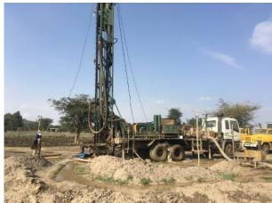
Preparatory field investigation (test borehole drilling) proposed and implemented as a result of this project
