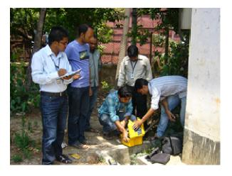
Leak detection using a mobile ultrasonic flow meter
