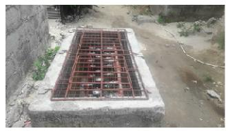
Manifold showing the water meters installed for house connection for ten households introduced by the phase 2 project (At Makadara area)
