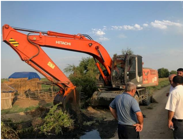
Working excavator with staff of AWF regional office and farmers (Aghjabadi)
