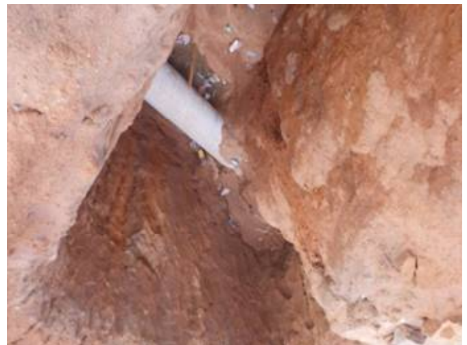
New Water Pipe at Chitungwiza
