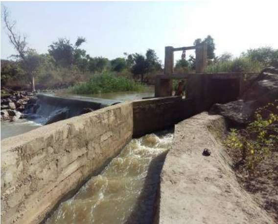
Sogido Small Scale Irrigation main canal constructed by the project
