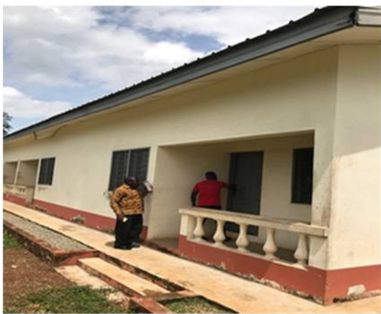
Teachers Bungalow Constructed at Krofofondo M.A. Primary Assin North District
