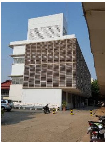
An exterior view of Lab Building
