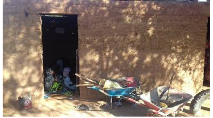
Classroom constructed by CGDES
