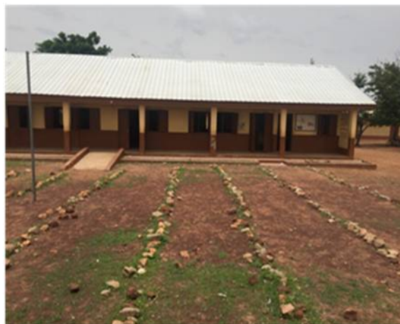
3-Unit Class Room block constructed at Samlimboukou B Primary School in the Bunkpurugu/Yunyoo District.
