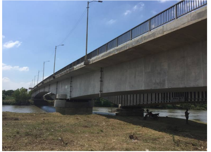
Led lamps above and river flow below the bridge
