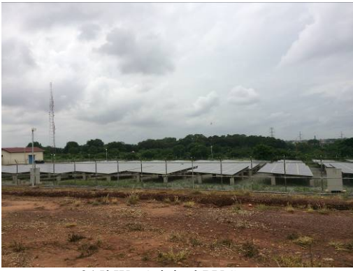
315kWp Original PV System
