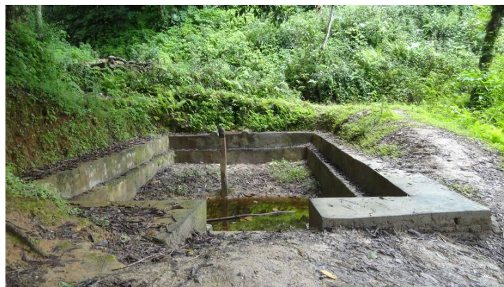
Water pond conservation at Paralmi, Gulmi district
