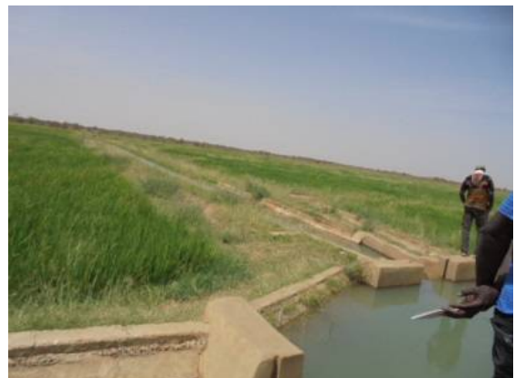
Small irrigation schemes rehabilitated in Podor (Podor 1)
