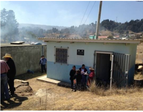
Groundwater supply facility of San José Chicalquix of Quetzaltenango
