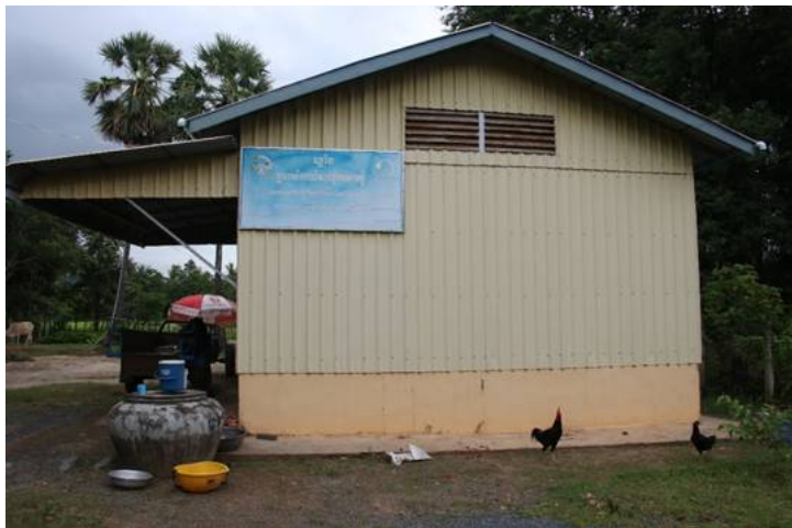
Warehouse of Phnom Touch Samaki SGG to store the produced seed (Banan District, Battambang Province)
