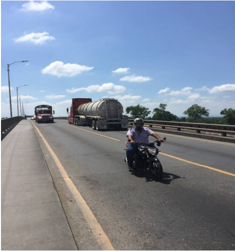
Commercial traffic going through the bridge
