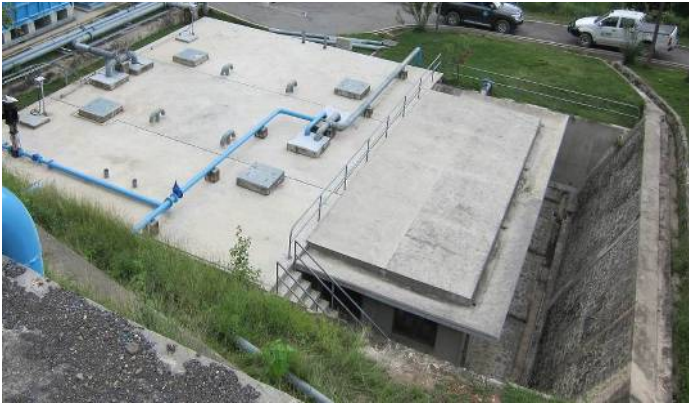
Lower Service Reservoir
