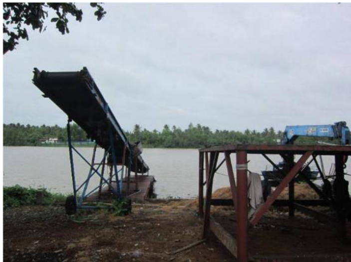
Proposed Project Site of Saline Intrusion Prevention Sluice Gate
