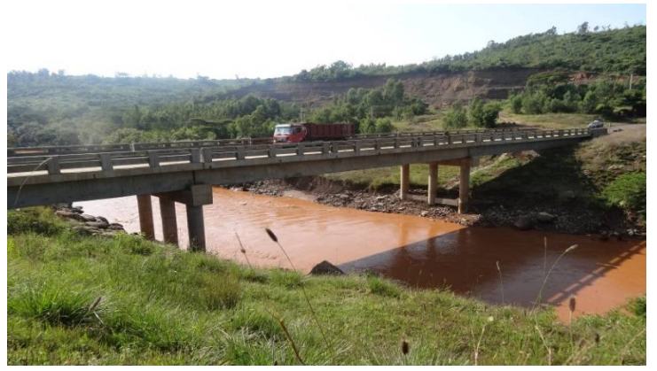
(Wabe Bridge in after replacement)
