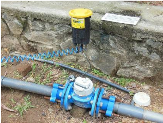
Checking the flow measurement in DMA 3 of Colombo City
