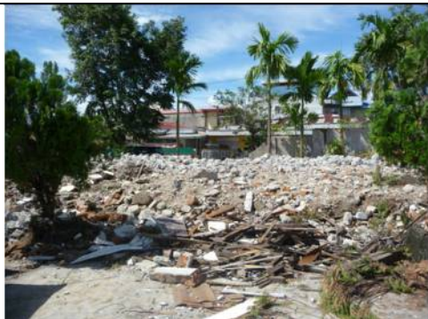
Before the project (December 2009)
