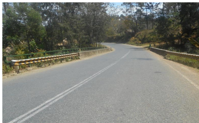
Orompaka bridge with two-track
