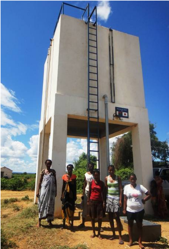
6 members of the water management committee of a pumping water supply system
