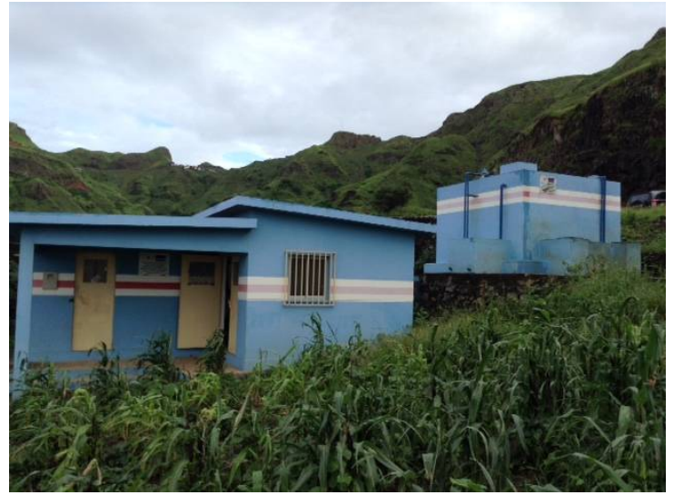
Water tank and machinery room in Levada (San Lorenzo dos Orgãos)
