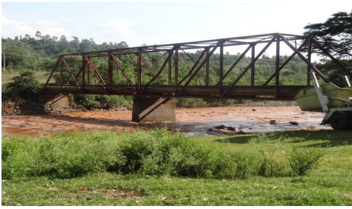
(Wabe Bridge in Southern Nation Nationalities and Peoples Region before replacement)
