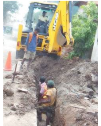
Old pipe replacement with new pipes in DMA9 in Colombo City
