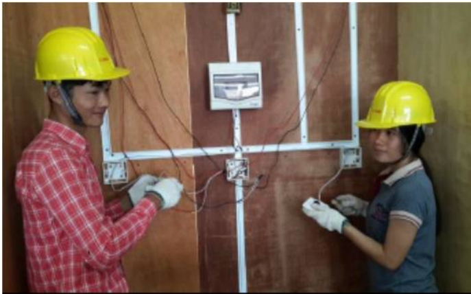
(Female and male participants in the training course on building electrical wiring)
