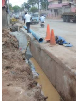
Old pipe replacement with new pipes in DMA9 in Colombo City
