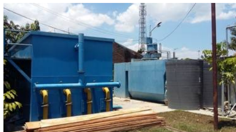
New reservoir and water treatment plant of PDAM Gowa
