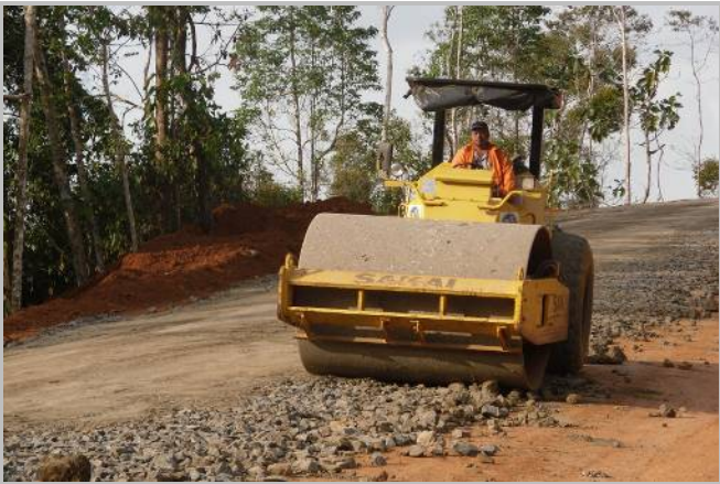
(Road improvement with the procured equipment)
