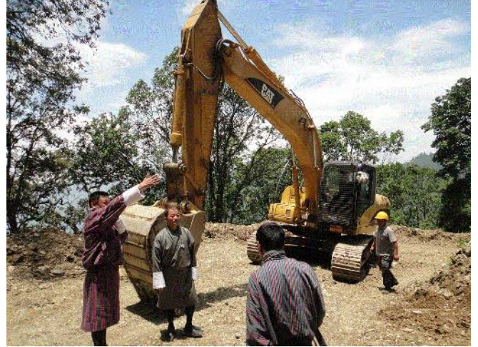
Farm road construction site
