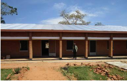
(A school block of two classrooms at Kalambwe primary school constructed as one of the DEP projects in Nkhata Bay District)
