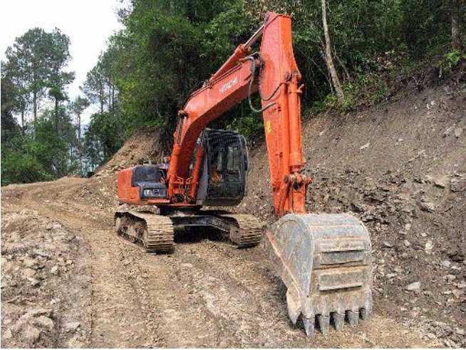
Farm road under construction
