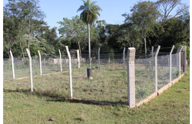
Yvaroty, La Colmena Municipality, Paraguari Province (One of the 25 prioritized villages) Construction of deep well: drilling of well and setting of casing (not setting of submersible motor pump)
