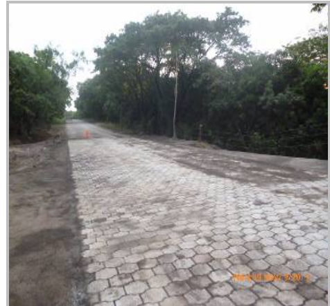
(Improved road after damages in the rainy season)
