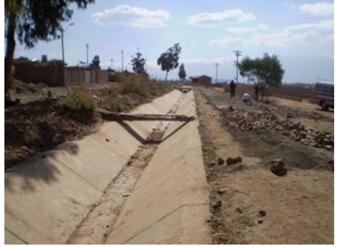
After the Project
