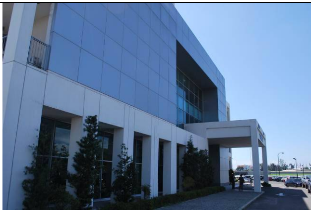
Exterior of the Center
