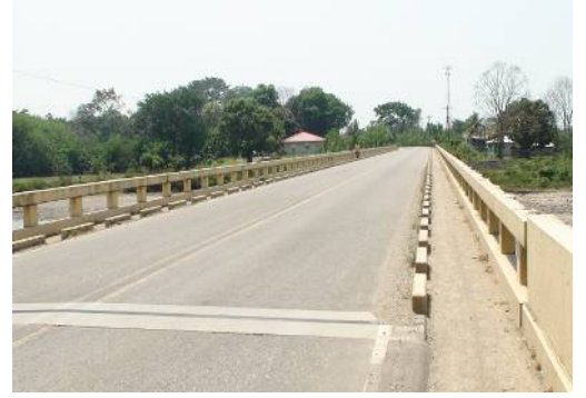
Superstructure(from the north)
