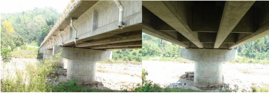
Superstructure: bridge support, bridge abutment (from El Progreso)
