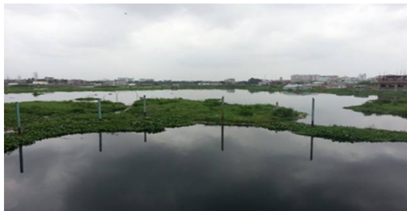
some part of the existing regulating pond some part of the existing regulating pond
