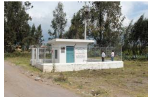
A well administration building constructed by the project
