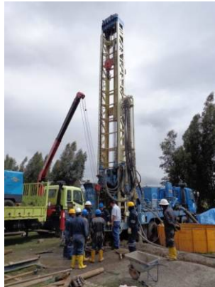
Drilling equipment procured by the project.
