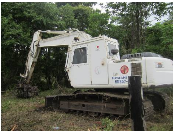
Brush Cutter cutting tree in a mine field in Banan district
