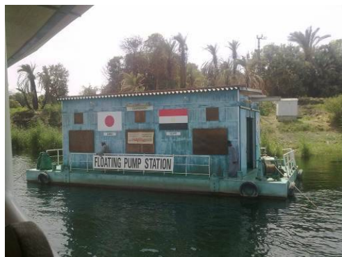
Floating Pump Station
