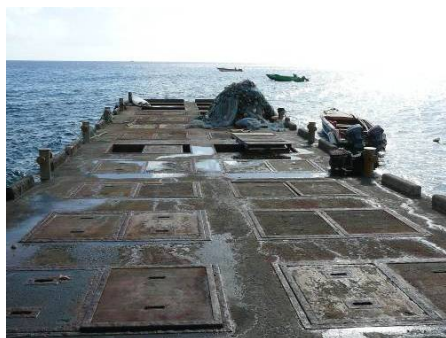
A fishery boat mooring at the west side of the jetty
