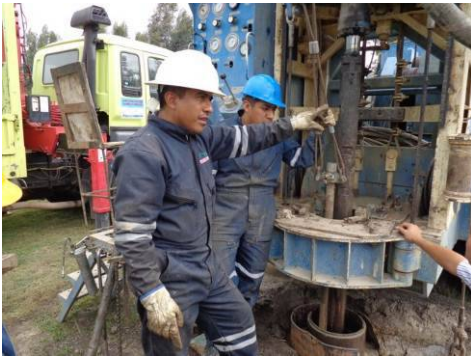
Engineers who gave instructions at a well drilling site.
