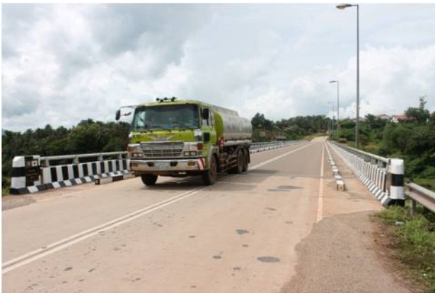
The new Hinheup bridge
