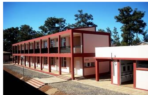
Dormitories constructed by the project
