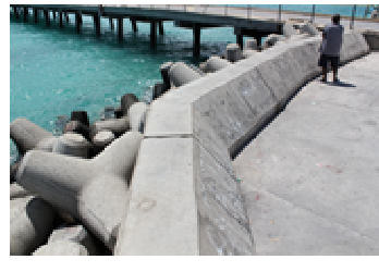
Current status of Fishery Jetty Revetment
