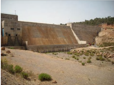
Concrete Dam (Ain Kawachia Dam)
