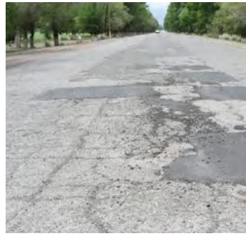
After the repair of BNT road (June 8, 2012)
