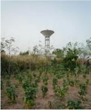
Water Tower constructed by the Project
