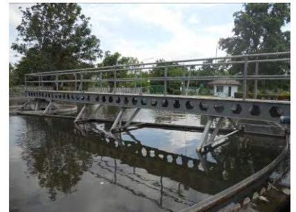
Clarifier Tank at STP
