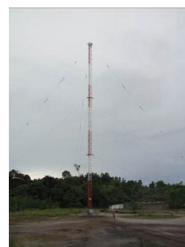
Medium wave transmission antenna
