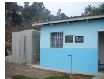
Pump station and water tank (Chimaltenango Department)
