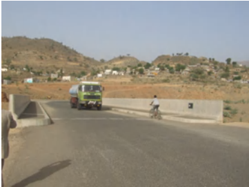
Gindae Bridge (new construction) and the bypass road
