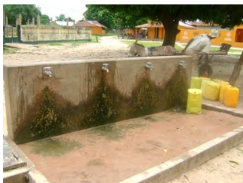
Public water tap in Fass
