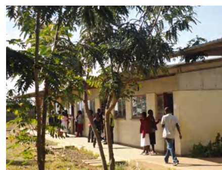
Students of the Cuamba IMAP and school building constructed by the Project
