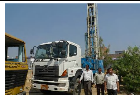
Using a drilling machine procured by the project
