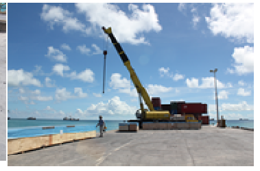
80t Truck Crane Truck in operation
