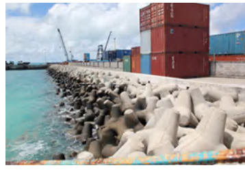
Current status of the New Wharf (North) after the project
