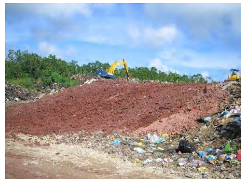
M-Dock Landfill in the cover soil operation
