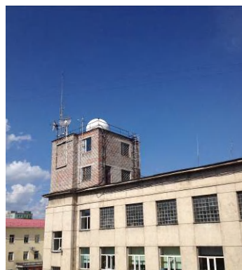
Receiving Facility of DDS Monitoring Data
