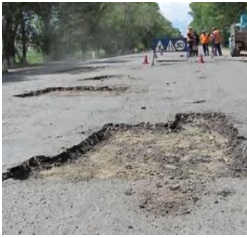
Repairing potholes of BNT road (June 5, 2012)
