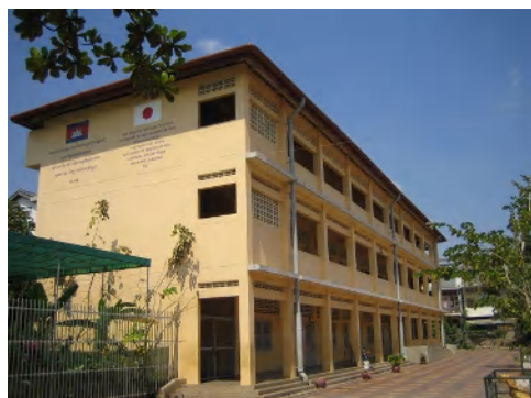
Side view of school building
