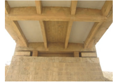
Baring of Emculu Bridge (repaired)
