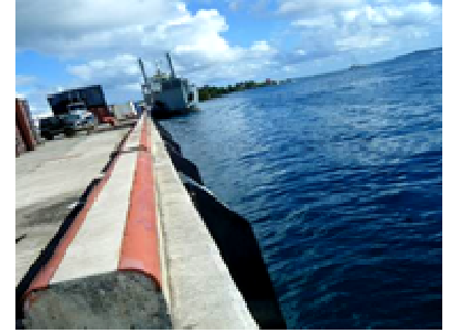
Current situation of Pier B, renovated by the project
