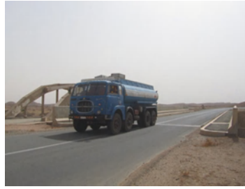
Dogali 2 Bridge (new construction) (existing bridge at the back)
