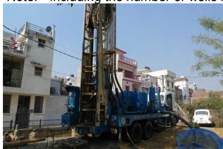
A well being drilled by project equipment
