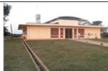
A hospital constructed by this project
