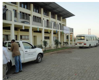
Well maintained administration building, mini-bus, official vehicle
