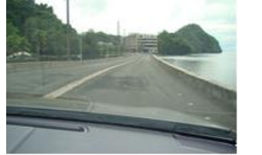
Malakal Causeway (After the renovation of pipe explosion)
