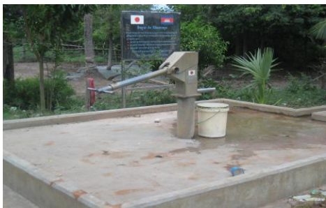
Japanese funded well in good condition with well maintained by the residents and providing safe water all year without dry up
