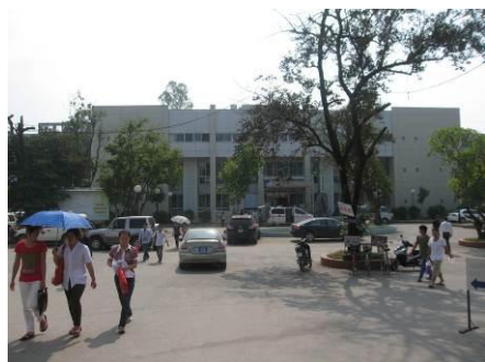
High Tech Block of Hoa Binh General Hospital
