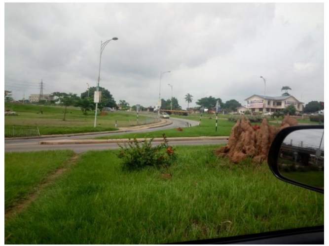
Asokwa Interchange linking the Middle Ring Road, Kumasi
