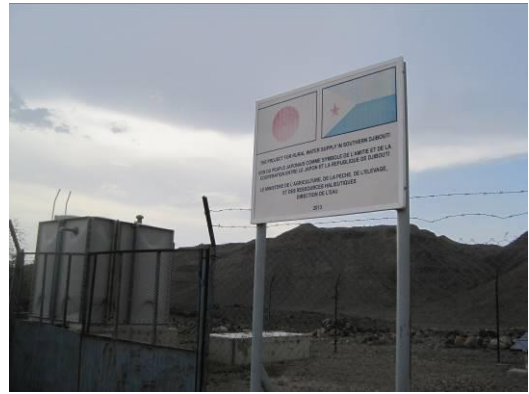
Sek Sabir water supply facility
