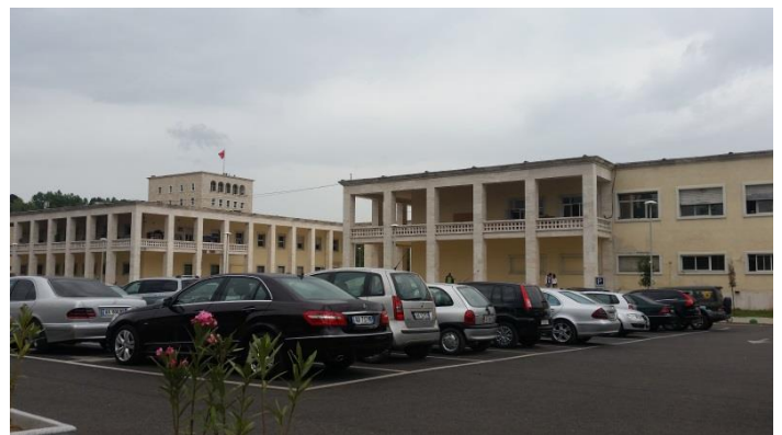
Newly Constructed Parking Facility in Tirana
