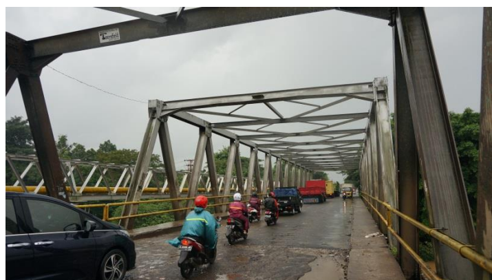
Pilot Project Site for bridge maintenance
