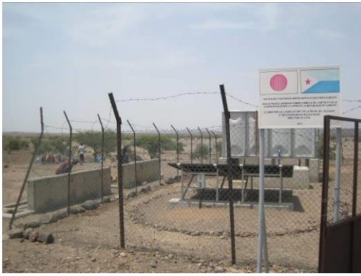
Afka Arraba water supply facility
