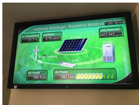
Display showing the amount of electricity generated etc. installed at the front entrance of the OI building
