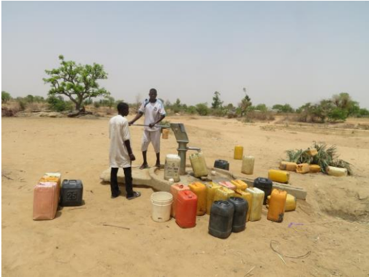
People fetching water at a borehole drilled using the rig procured under the project in Katsina
