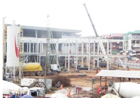
Construction of Kejetia Terminal Complex, Kumasi
