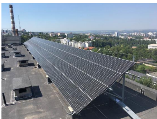
PV modules installed on the roof of the building of OI
