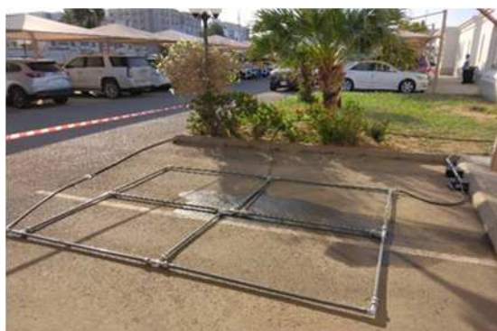
Photo 3 Imitating piping network
