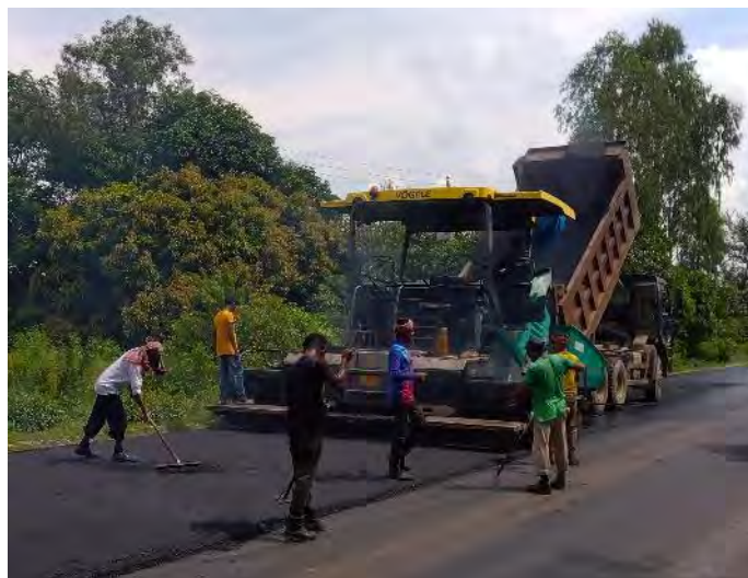
Figure 2.7.3 Overlay Repair Work on National Highway No.1
