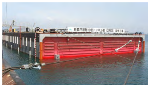
Figure 2.7.11 Sandwich-structured Immersed Tunnel
