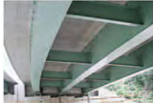
Figure 2.7.9 Steel Narrow Box Girder Bridge
