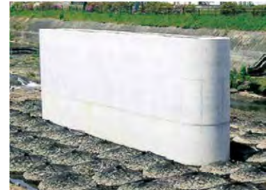
Figure 2.7.14 Bag Materials for Scour-Prevention Bag-Type Rooting Method
