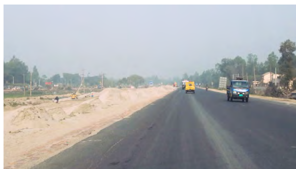
N4 (Elega - Jamuna Bridge) Under Construction
