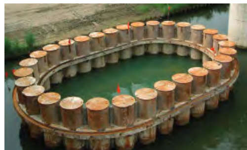
Figure 2.7.7 Steel Pipe Sheet Pile (SPSP)
