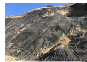
Netting installed on a road controlled by the Indian
