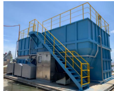
Installation work completed
