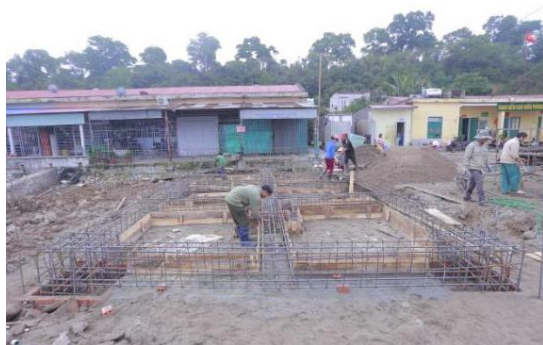
Reinforcing bar assembly
