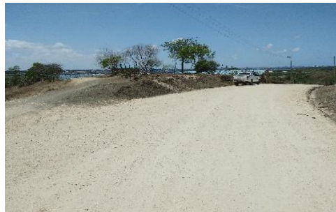
Photo 1 Power grid laid on the road
