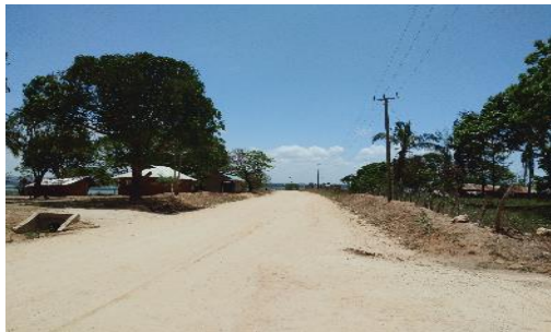
Photo 4 : Near the junction (Near candidate sections 3 and 4)
