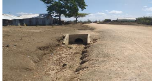
Photo 3 Drainage system for existing main road
