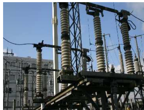
Disconnection Switch
