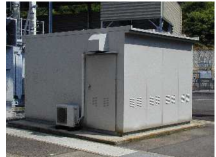
Metal-clad switch gear
