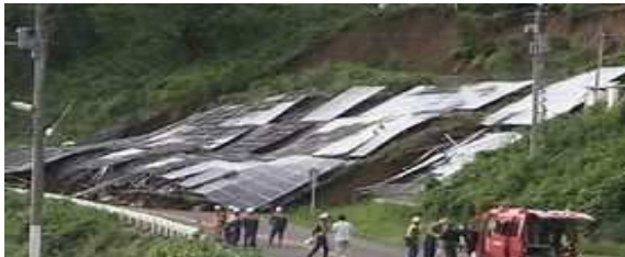
An example a landslide caused by flood
