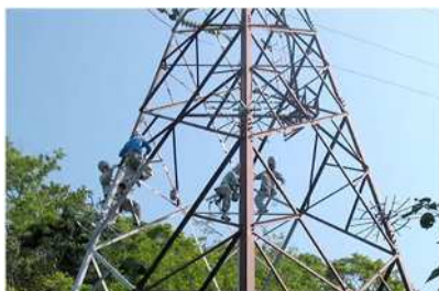
https://www.chuden-kogyo.co.jp/works/painting.html Rust-proof painting of steel tower
