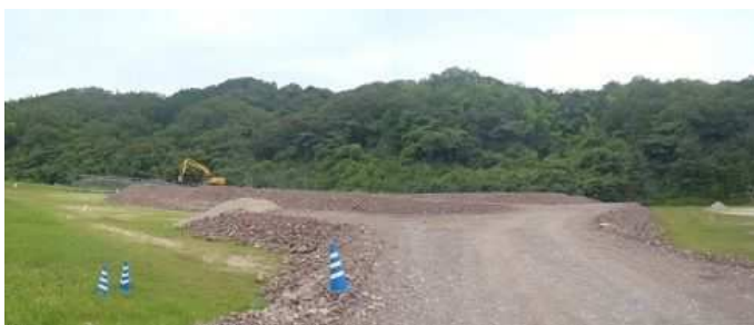
Construction of access road
