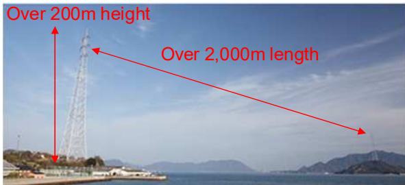
Transmission lines across the sea in Japan
