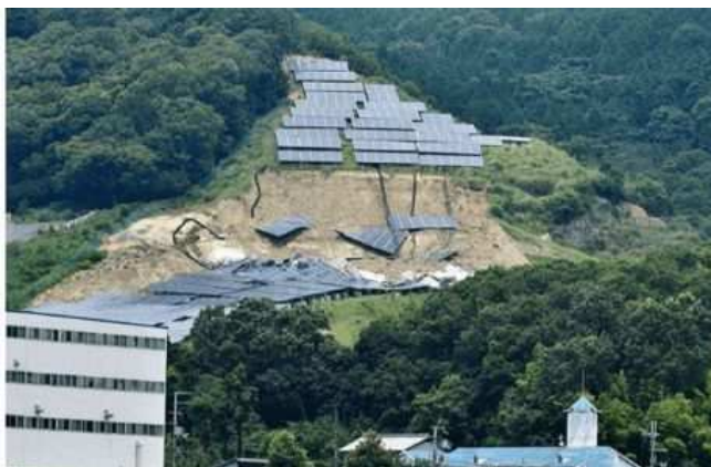
An example of a landslide caused by an earthquake
