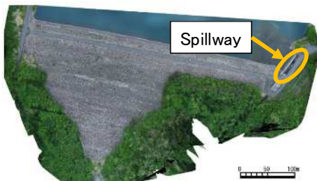
Spillway installed near the dam body
