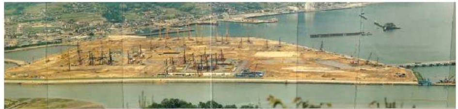
Photo. Site preparation (view from west side)
