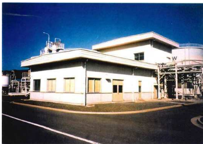
Photo. Wastewater treatment facility
