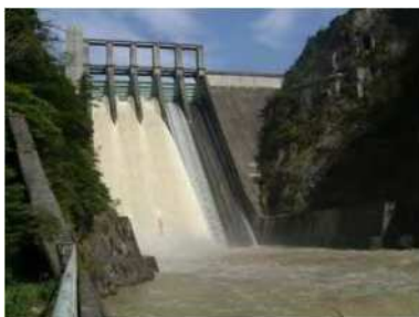
Spillways with gates
