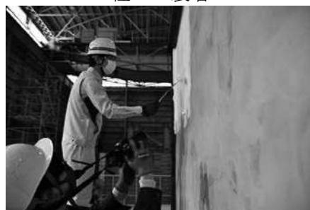
Power Coating 1回目の塗布
