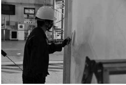
Power Coating 2 回目の塗布
