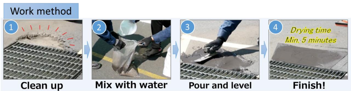
Figure 2: RockMor work method
