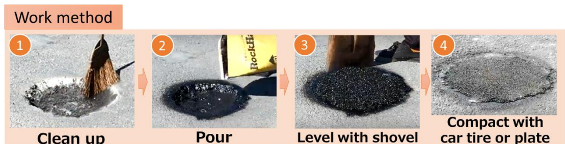
Figure 3: RockHard work method
