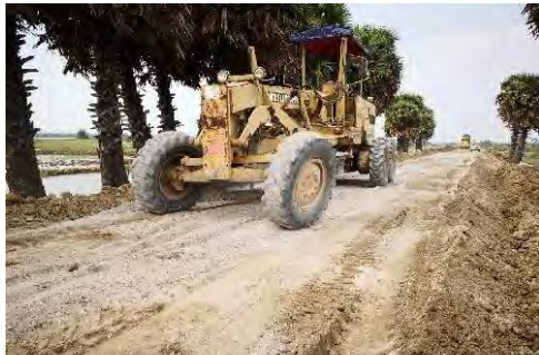
Sub-base was spread evenly, levelled and compacted
