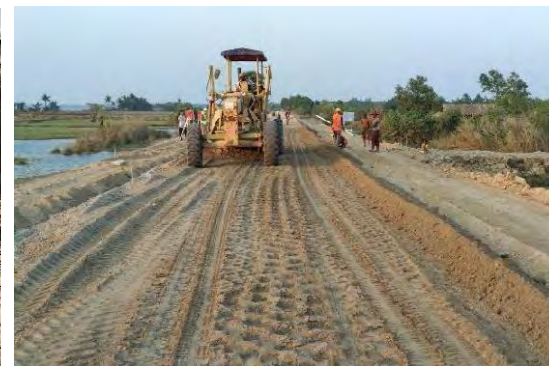
③ Subgrade/ Capping layer construction work
