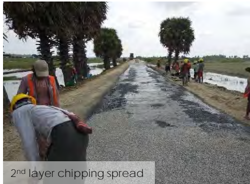
2nd layer (finishing coat) done
