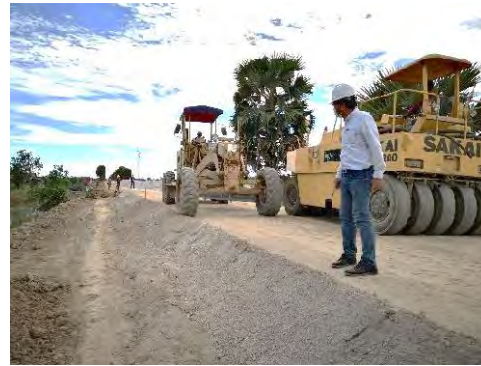
Sub-Base course compaction done
