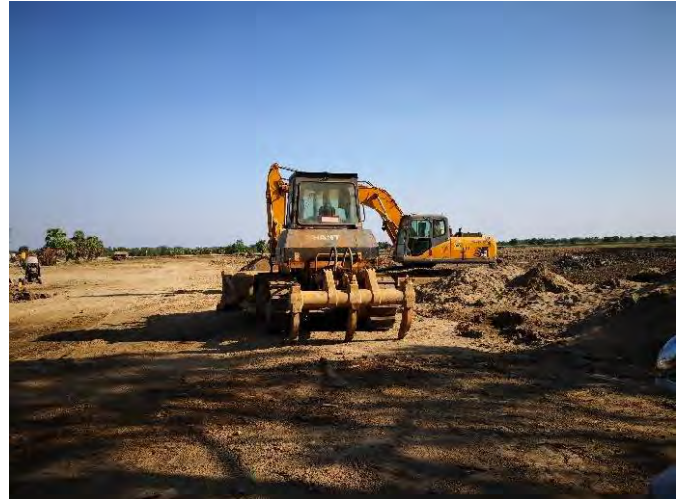
MOC machines allocated on site for construction
