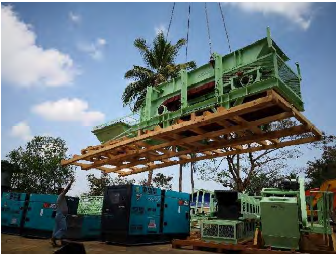
WSF feeder unloaded
