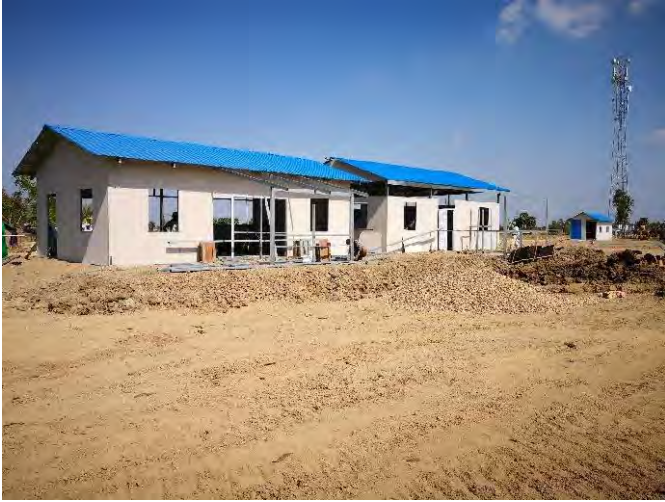
MOC site office (left) and JDC site office (right)
