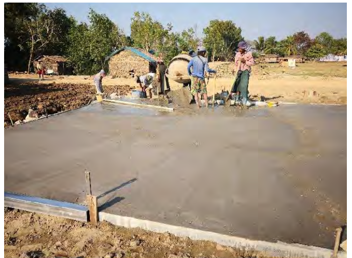
Slab concreting for JDC site office
