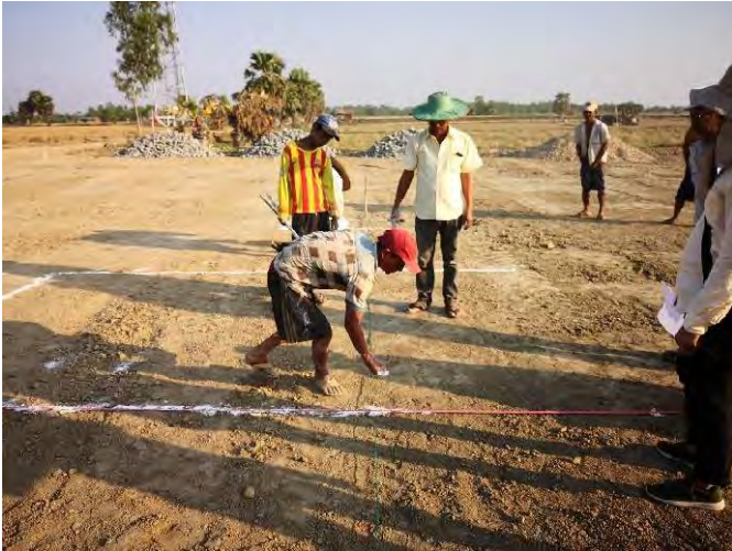
Measurement and chalk marking by MOC-JDC
