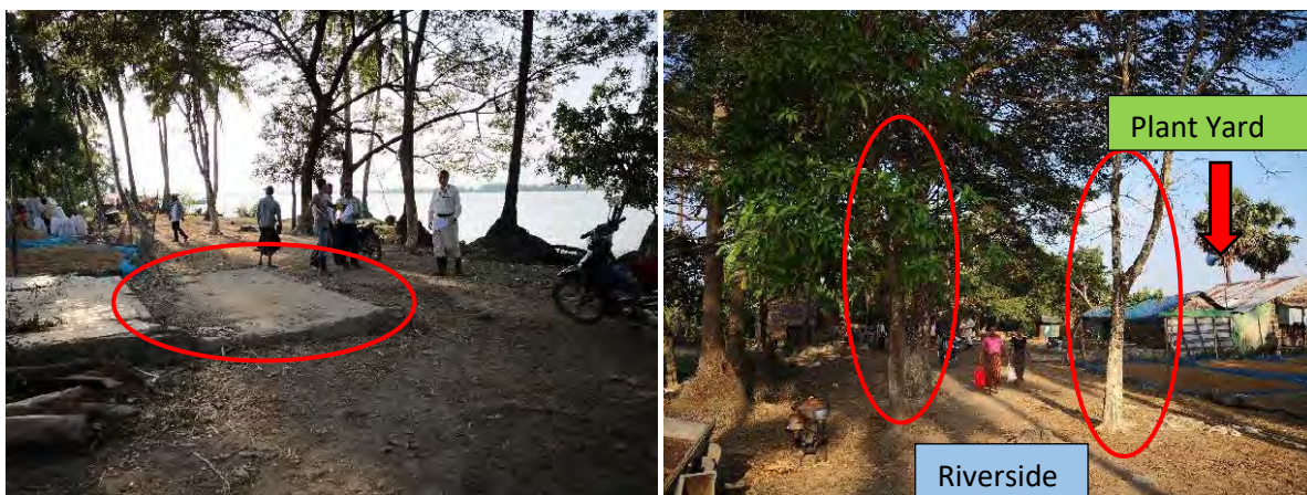
Existing RC slab and trees along the access from riverside to plant yard to be removed.
