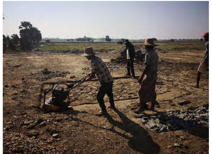
Compaction to be carried out before concreting
