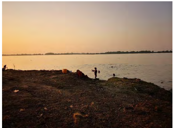
Jetty clearance done
