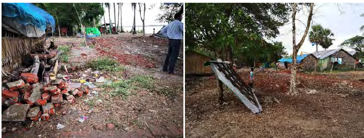
Existing brick slab was removed; trees obstructing the access to be removed shortly.
