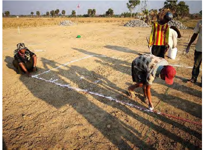
Measurement and chalk marking by MOC-JDC
