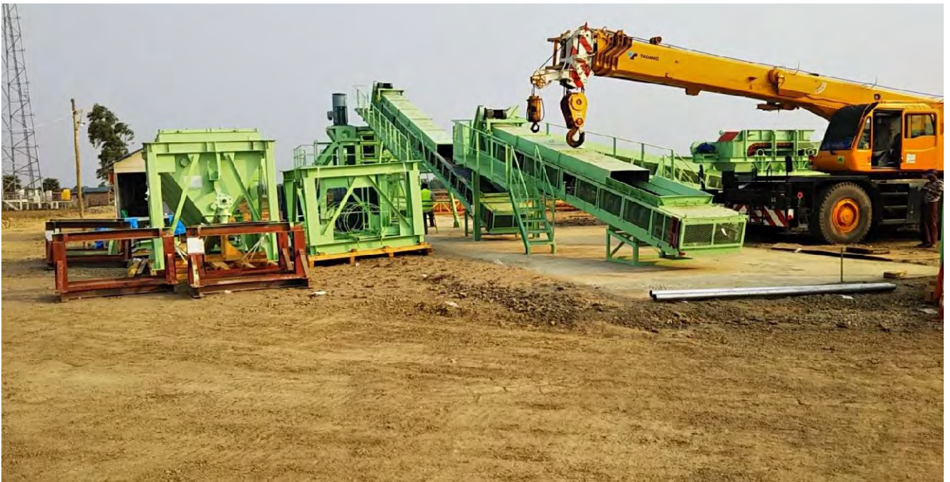
Placement of Belt Conveyer-1 (BC1) & Belt Conveyer-2 (BC2) in position done
