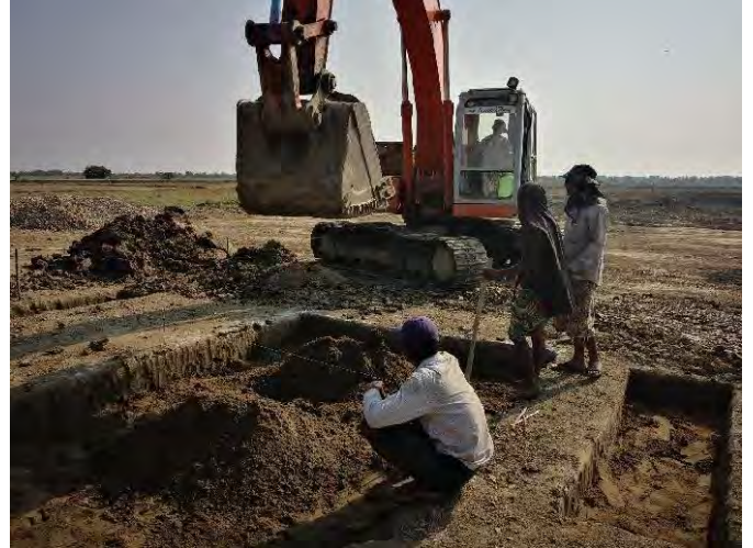
Soil levelling of slab foundation
