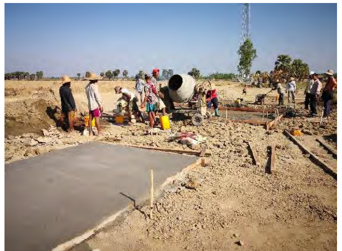
Part of slabs done concreting and continue for next slab
