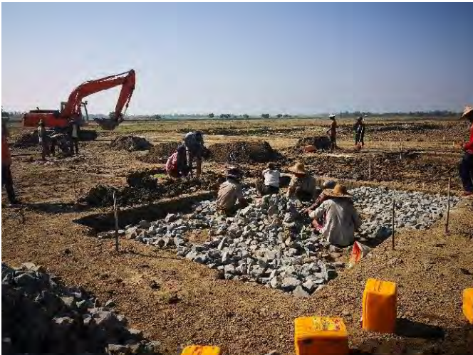
Laying hardcore for the slab foundation
