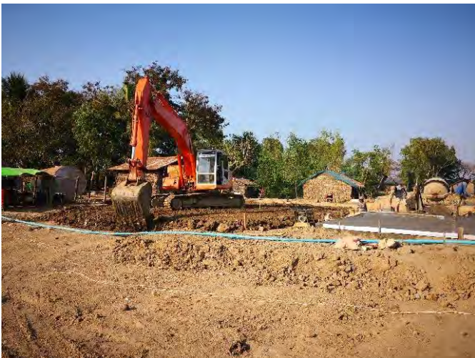
Soil levelling for MOC site office
