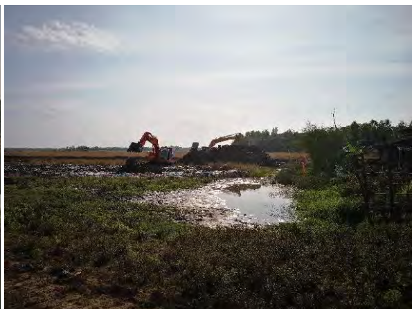
Earth bunds were erected by excavators to indicate site boundary.
