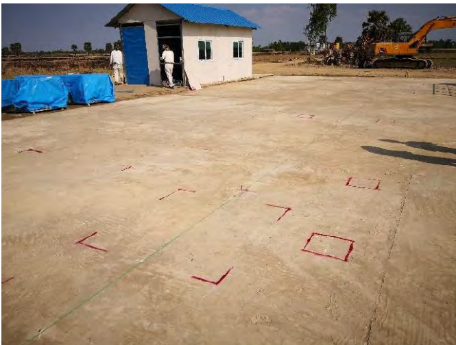
Equipments base and footing marking done
