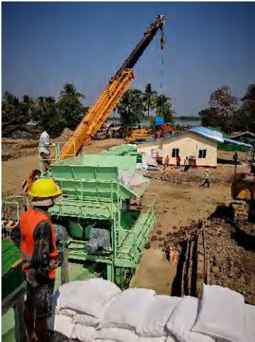
Preparation of machinery, material (lime), crane scale, perforated PVC pipe, ton bag
