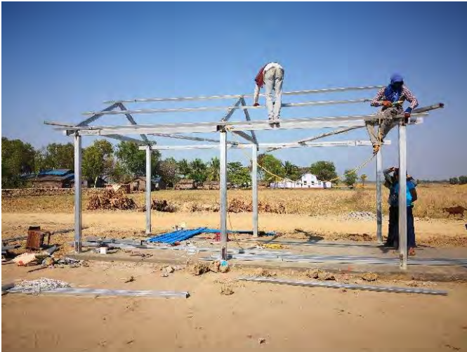
Erection of control room in progress (AM)
