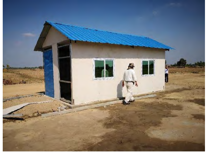
Exterior of control room
