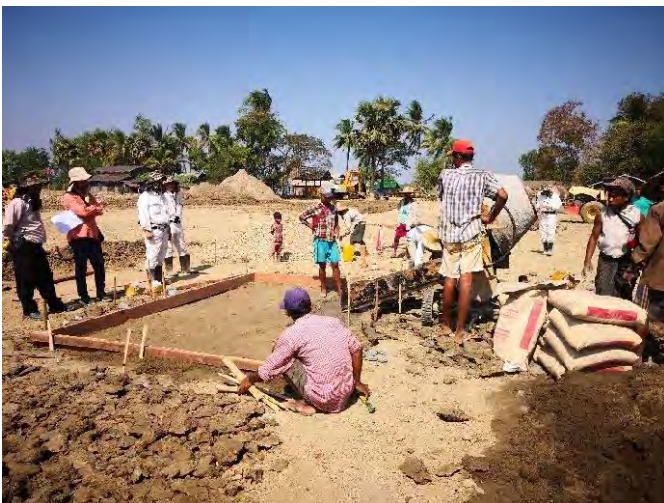
Concreting start after formwork erected
