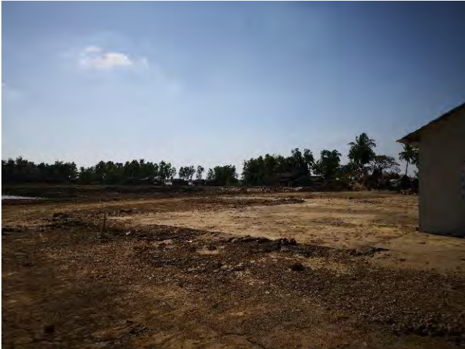
Twister machine yard RC slab completed
