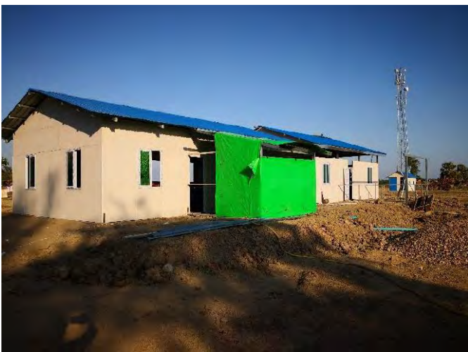
MOC office toilet erection works ongoing
