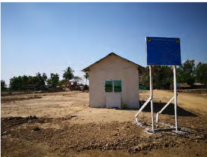
Control room next to Twister yard (site)
