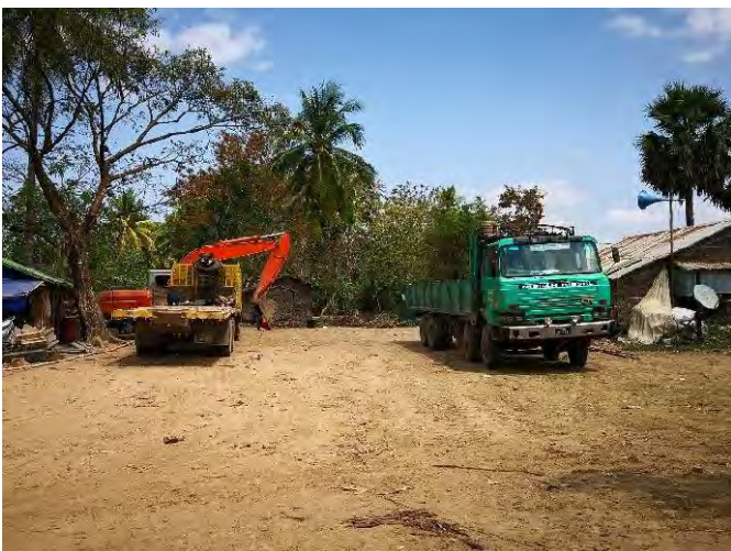
10 ton Trucks standby at site for transportation
