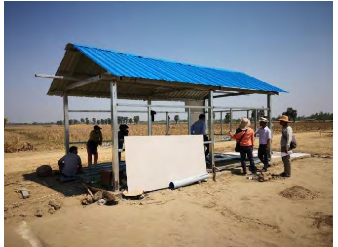
Erection of control room in progress (PM)
