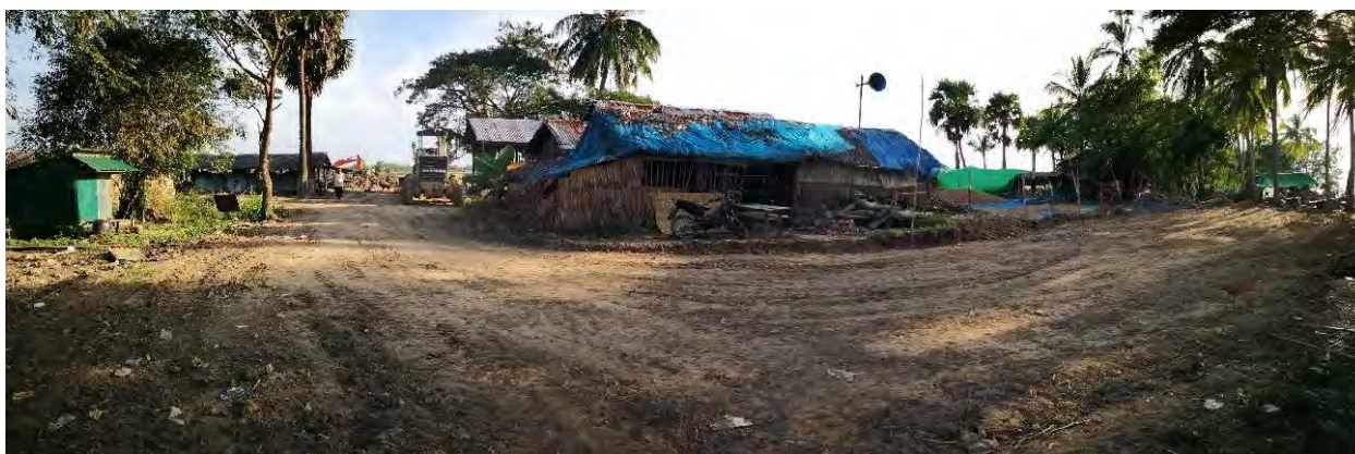
Existing access road from riverside to plant yard was widened and made good by MOC
