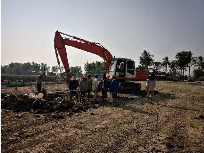
Excavation of Twister foundation
