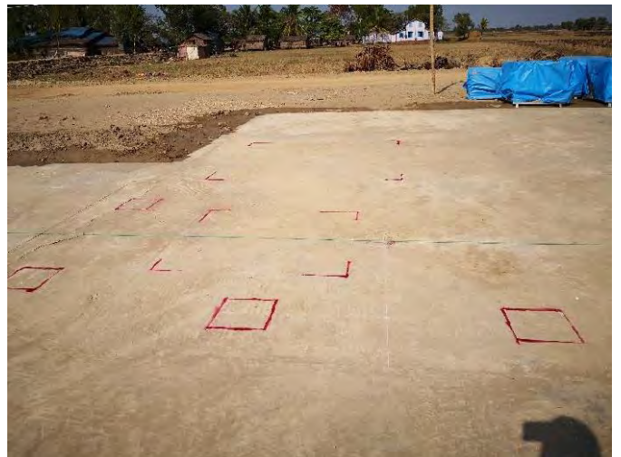
Equipments base and footing marking done
