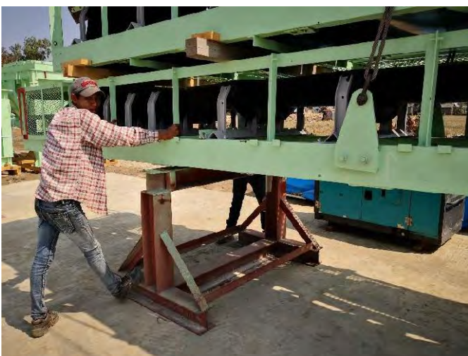
Adjustment on BC3 stand to stabilize BC3 placement
