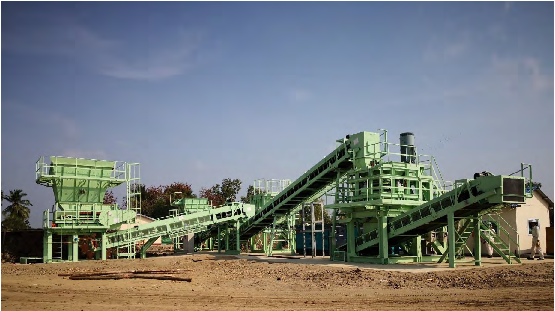
Assembly, Testing and Commissioning of Twister Plant Completed...
