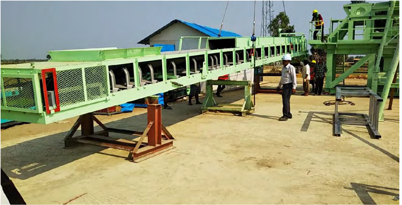
Placement of Twister Belt Conveyor-3 (BC3) in position done
