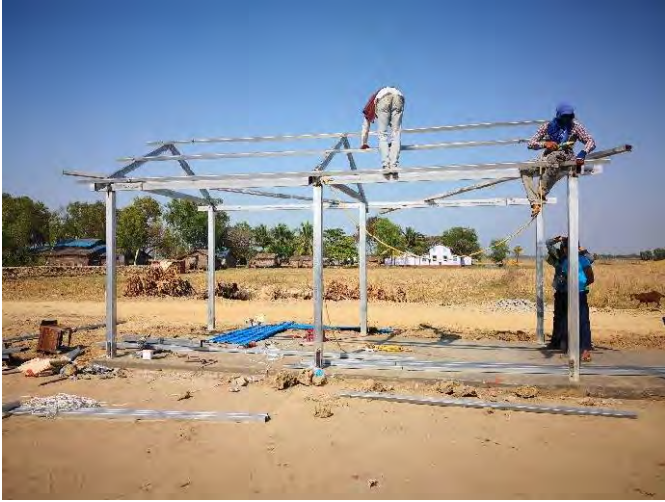
Erection of control room in progress (AM)
