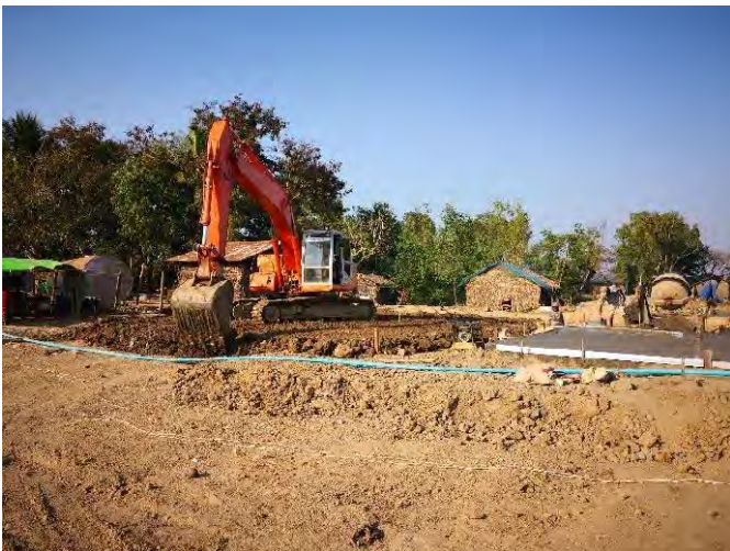
Soil levelling for MOC site office
