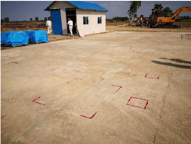
Equipments base and footing marking done
