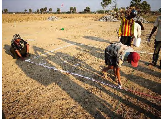
Measurement and chalk marking by MOC-JDC
