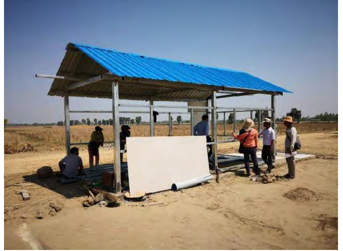
Erection of control room in progress (PM)
