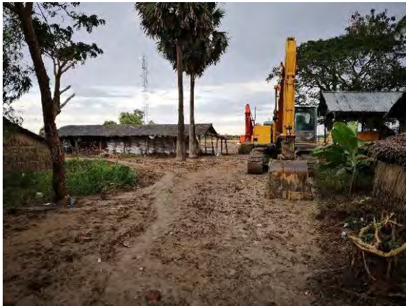
Existing access road from riverside to plant yard was widened and made good by MOC.
