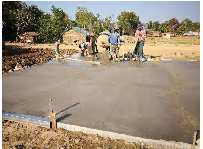
Slab concreting for JDC site office
