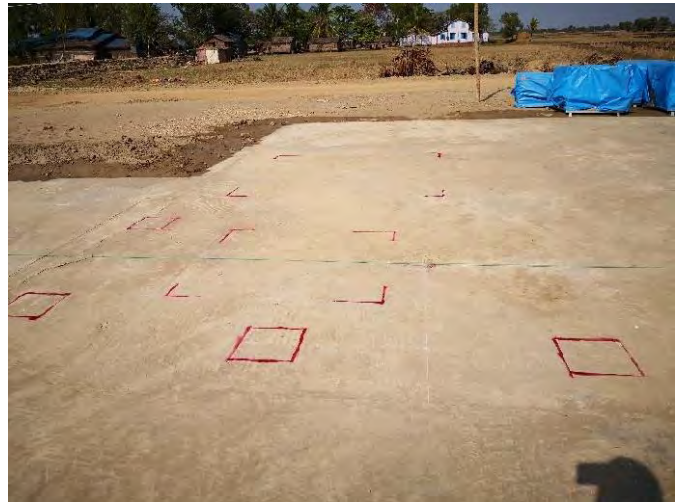
Equipments base and footing marking done
