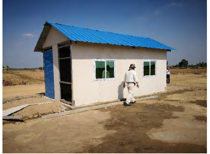
Exterior of control room
