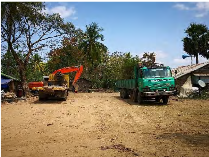
10 ton Trucks standby at site for transportation
