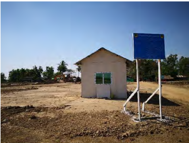
Control room next to Twister yard (site)
