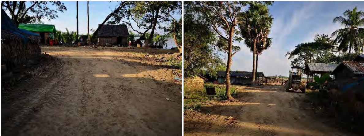
Existing access road from riverside to plant yard was widened and made good by MOC
