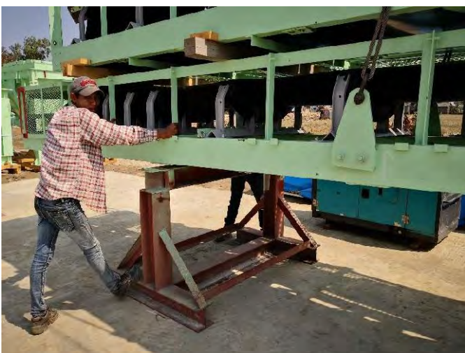
Adjustment on BC3 stand to stabilize BC3 placement
