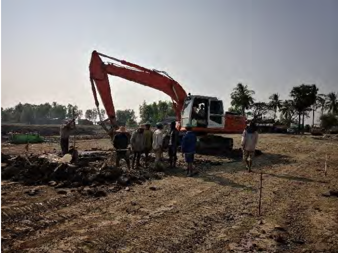
Excavation of Twister foundation
