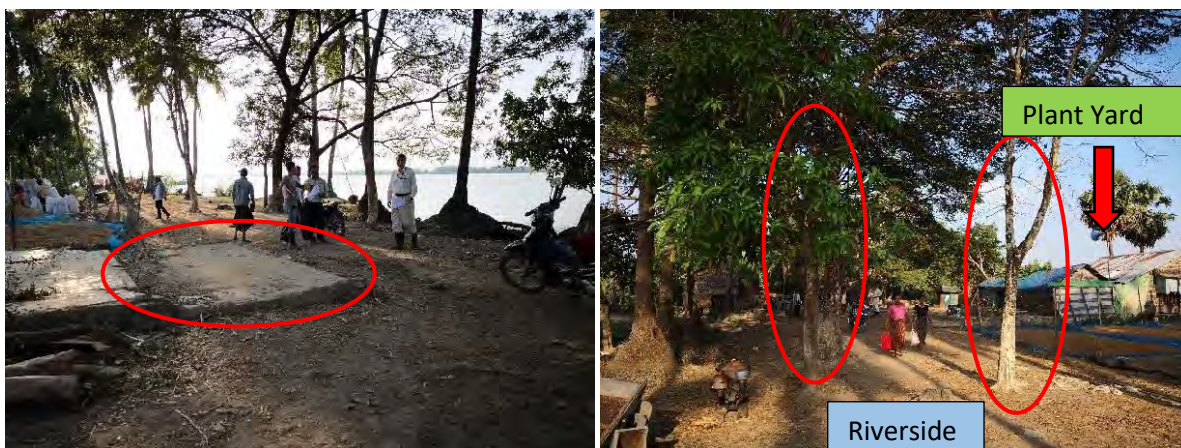
Existing RC slab and trees along the access from riverside to plant yard to be removed.
