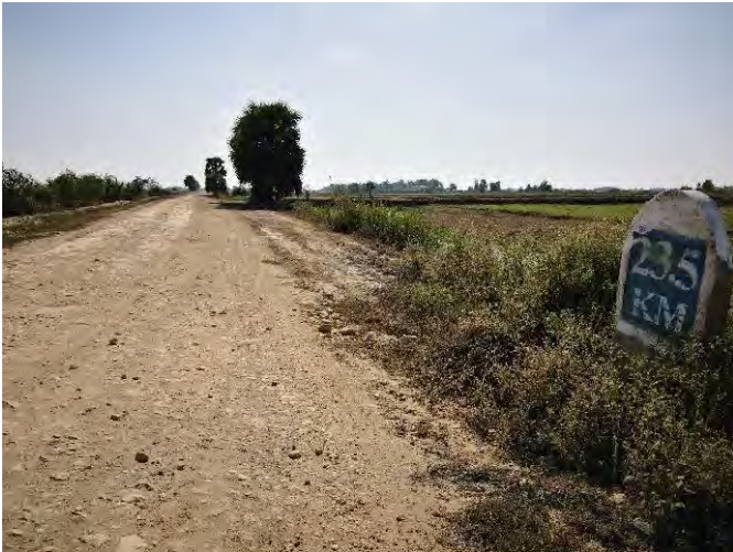
Beginning of test section (23.50km)
