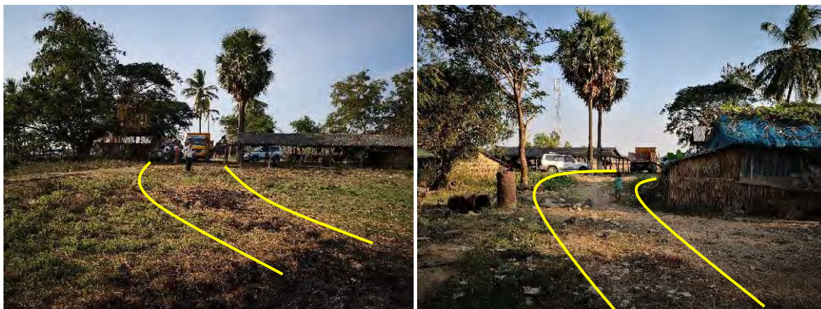
Existing access road from riverside to plant yard to be made good by MOC.
