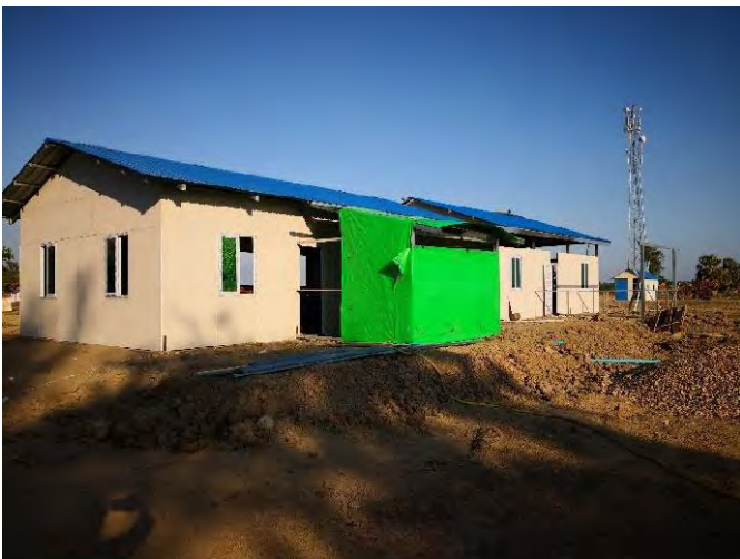
MOC office toilet erection works ongoing
