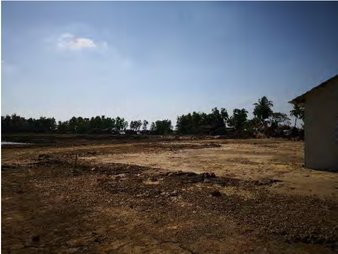
Twister machine yard RC slab completed
