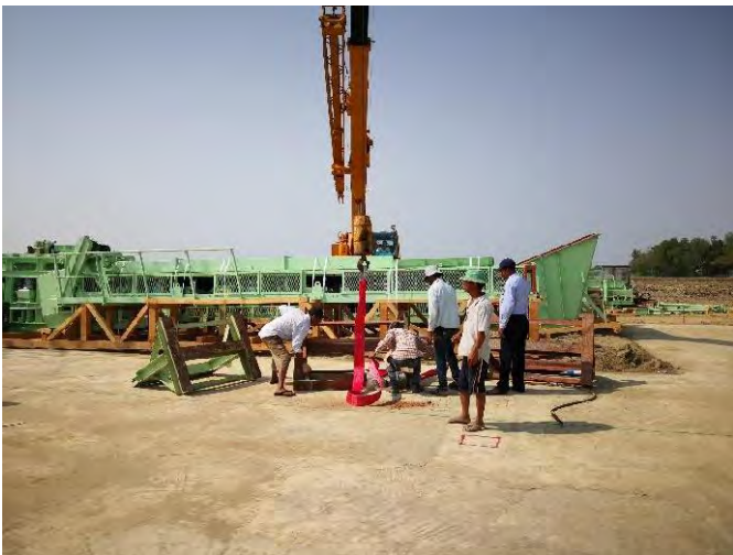
Setting of BC3 stand on particular locations (3 nos)
