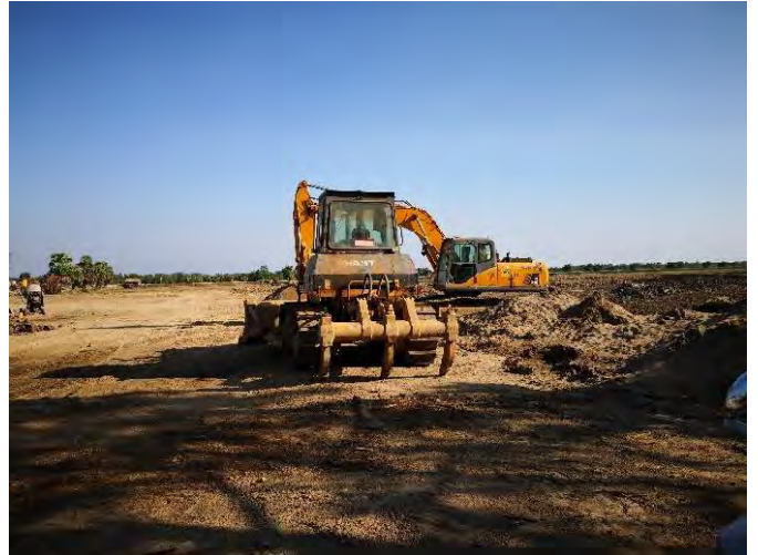
MOC machines allocated on site for construction
