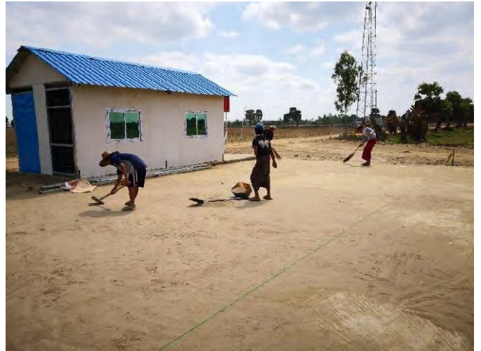
Cleaning of plant yard for equipment marking works
