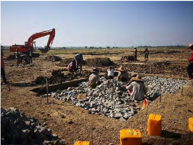
Laying hardcore for the slab foundation
