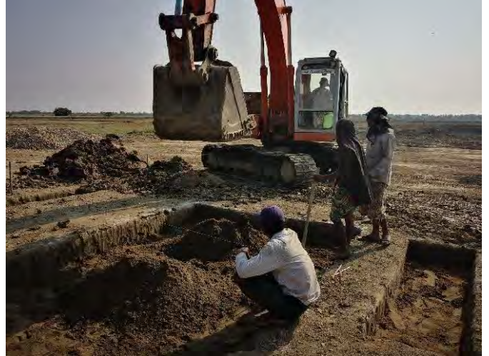
Soil levelling of slab foundation
