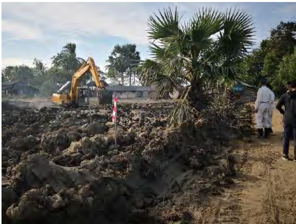
Excavators were stockpiling the clay soil to level the plant yard with access road.
