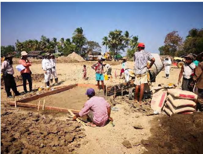
Concreting start after formwork erected
