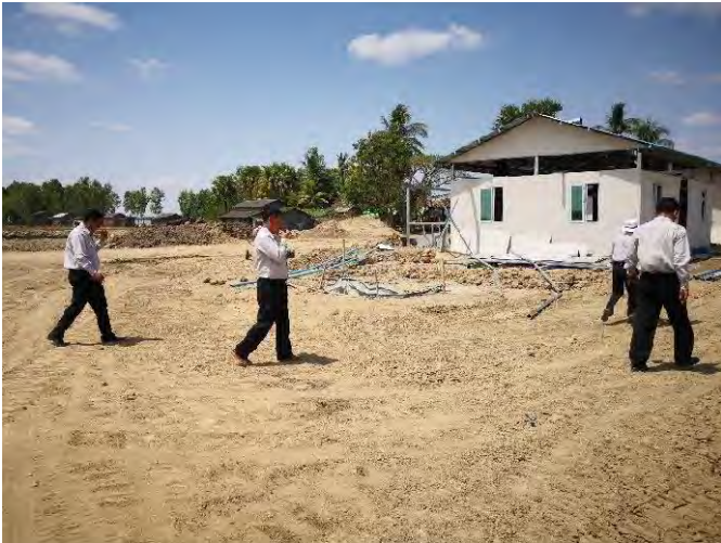
Site visit by MOC Chief Engineer, U Khin Zaw
