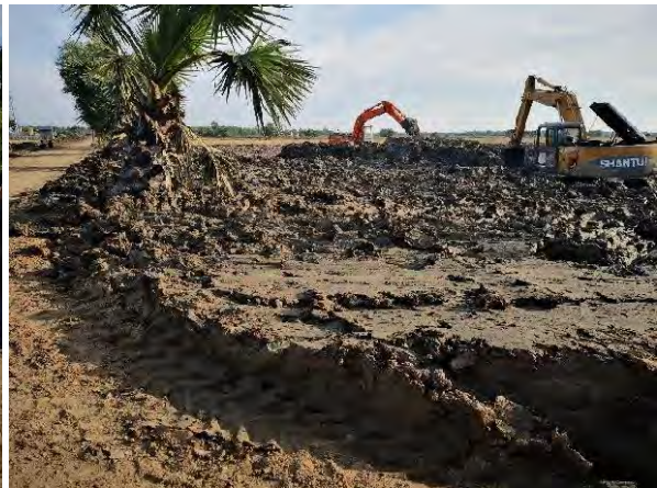
Excavators were stockpiling the clay soil to level the plant yard with access road.
