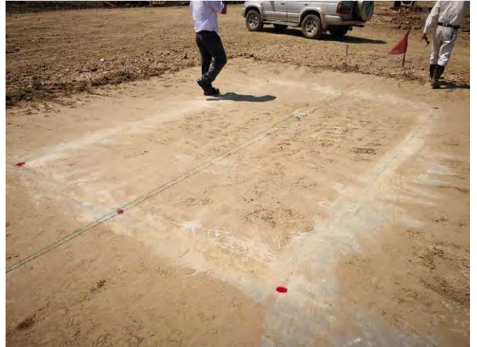
Joint measurement and marking of equipment location by JDC-MOC
