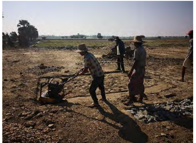
Compaction to be carried out before concreting
