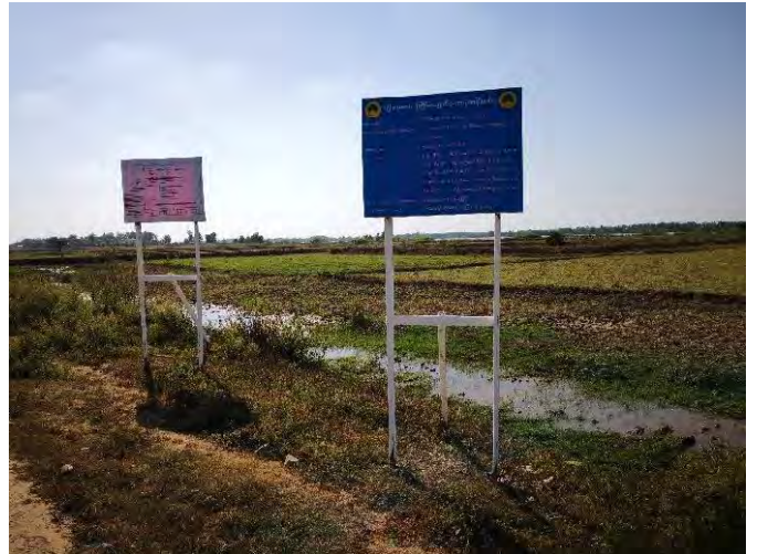
Construction site information board (23.50km)
