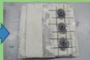
INSTALLATION OF ATTACHEMENTS AND CUTTING OF PERIMETER
