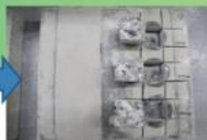
CONCRETE SUBSTRATE FAILURE
