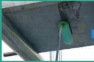
APPLICATION OF ALPHATEC 380S
