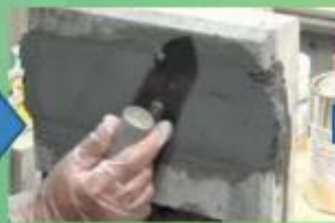
APPLICATION OF ALPHA PCM USING TROWEL
