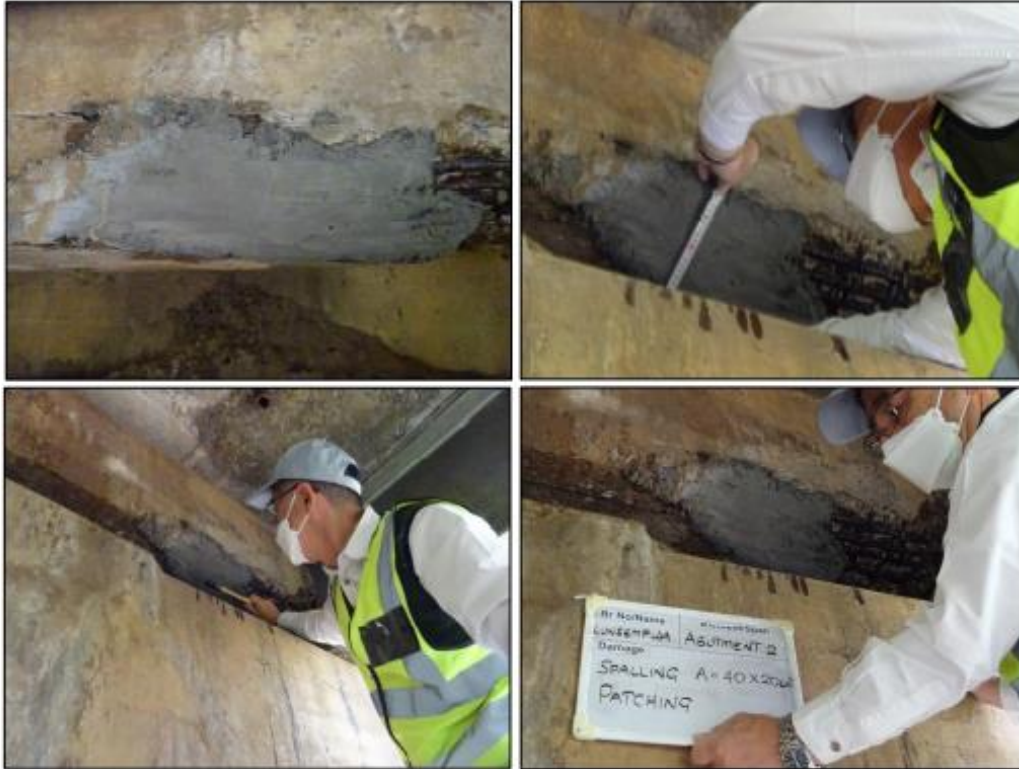
Photo 3: shows the condition of the Patching repair
