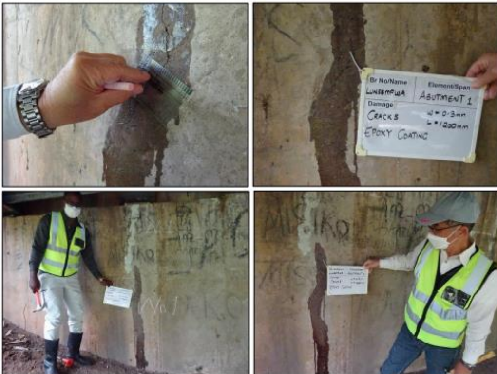
Photo 1: shows the condition of the Coating repair
