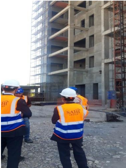
KRG-MOLSA conducts Occupational Inspections on construction projects in Erbil city in 2021
