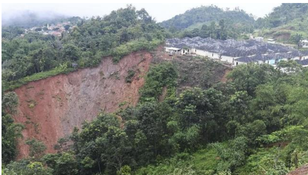
Figure 7-3 Example of slope failure
