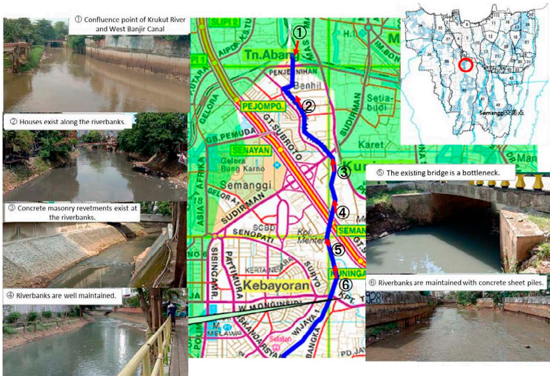
Figure 4-49 Current Situation in Krukut River Downstream (October 2021)
