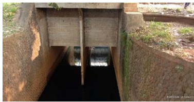
Existing Box Culvert
