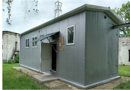
Photo 2: Exterior of pellet boiler building (Branesti)
