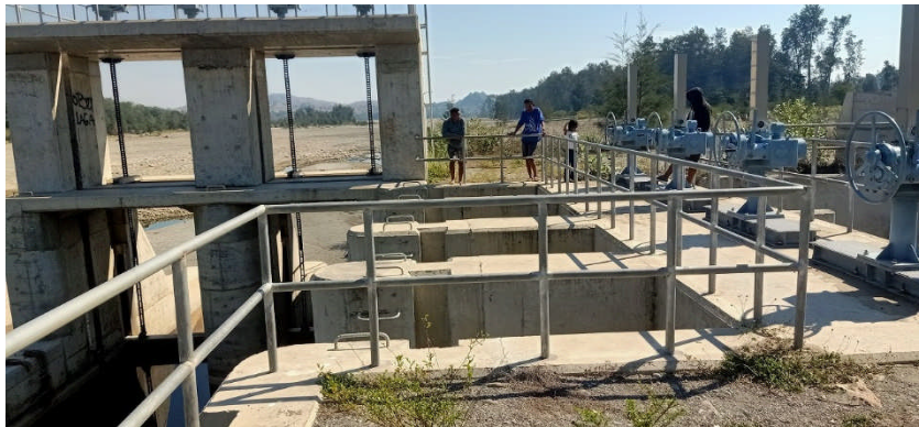
Photo 3: Irrigation facility developed by this project (Weir)
