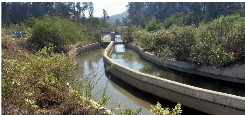
Photo 2: Irrigation facility developed by this project (Main canal) (2)
