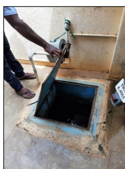
Underground Water Storage Tank
