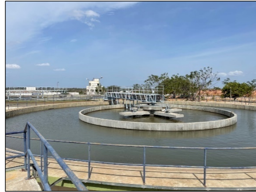
Water Purification Facility constructed by the Project (Thoothukudi)
