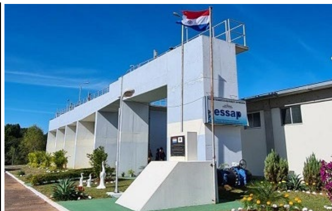
WTP Constructed under the Project
