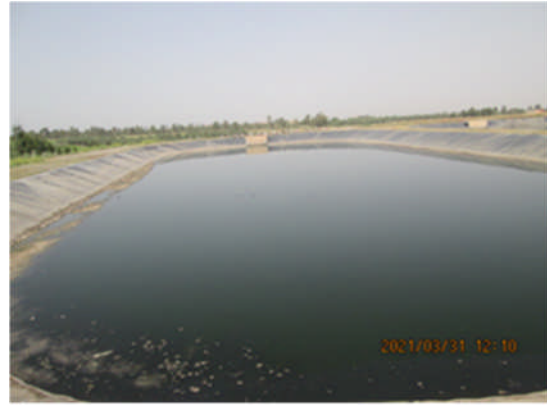
Sewage treatment facility developed by this project (Amizmiz City)
