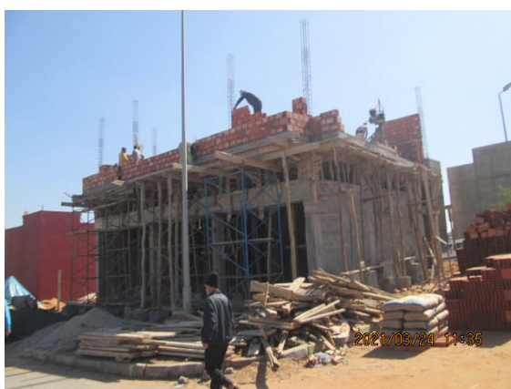
Photo 3: House under construction
