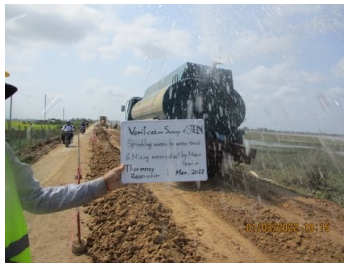
Sprinkle water by a water truck
