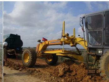
Agitate soil by a motor grader
