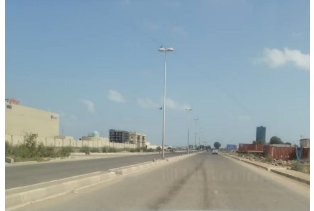
Photo 2: Road in Djibouti City, Developed by Utilization of the Road Maintenance Equipment
