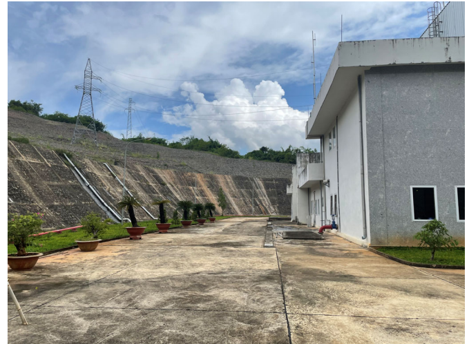
Exterior of the Thac Mo Hydropower Station
