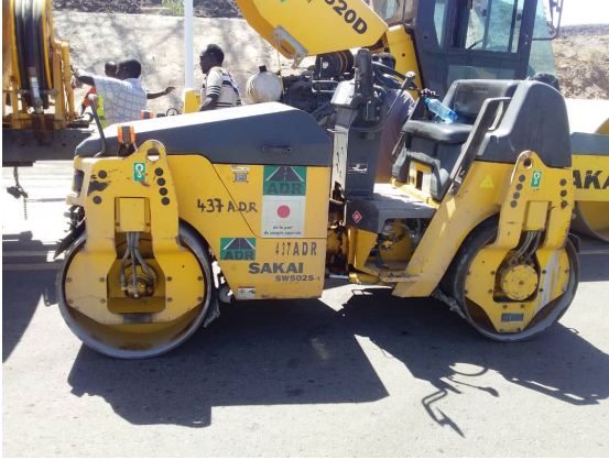
Photo 1: Procured Road Maintenance Equipment (Road Roller)
