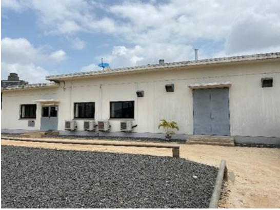
Control building (Ilala substation)
