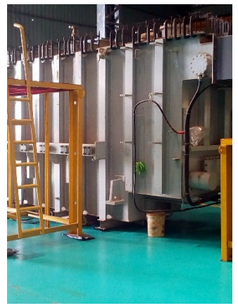
Transformer under repair
