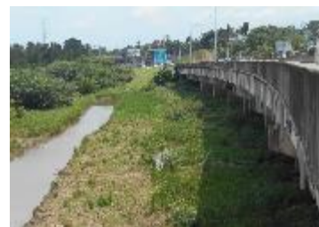
Viaduct built near the Kelani River
