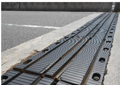
Expansion joint in the project section
