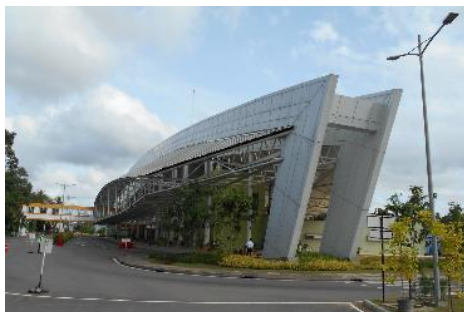
Exterior view of the MMC
