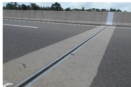
Expansion joint in other sections
