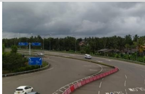
View near the Kottawa interchange
