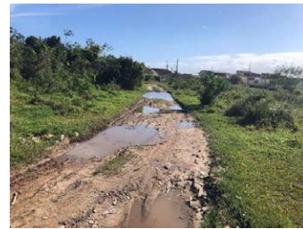
Figure 16 - Difficulty of access due to flooding shown in the picture
